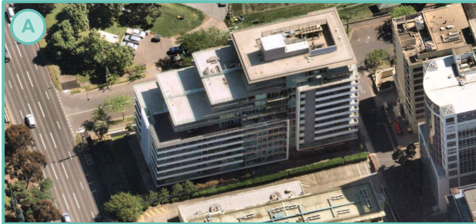
Picture 1: 48 Queens Road, viewing north
