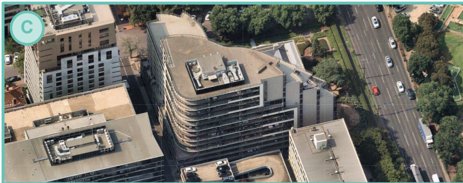
Picture 6 54 Queens Road, Viewing South
