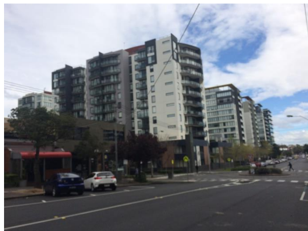
Picture 7 View east towards 148 Wells Street
