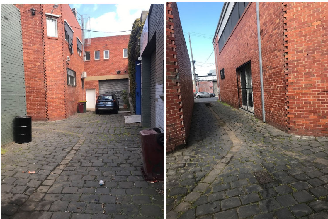
Figure 17: Argyle Place runs north off Thistlethwaite between Montague and Boundary streets. It is unusual because of its 'T' shaped configuration. The 1895 MMBW survey records that there were four cottages at the end of the lane, piggy backing four cottages with a frontage to Thistlethwaite Street. Source: Trethowan Architecture, 2020.
