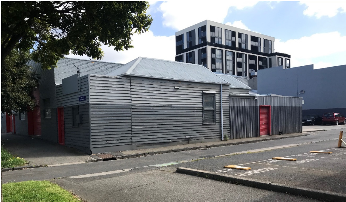
Figure 10: Former house in Buckhurst Street on the corner with Wilson Place. Source: Trethowan Architecture, 2020.
