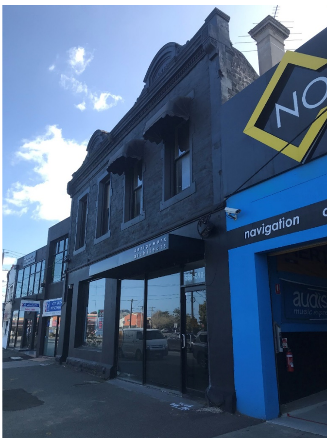
Figure 23: View of the pair of shops at 588-590 City Road. The building is well constructed with bluestone walls and rendered mouldings and could be regarded as perhaps the finest of the nineteenth century building lining the Montague section of City Road. The parapet records the construction date of 1879, relatively early in the context of the development of Montague. In 1895 the Sands and MacDougall Directory records that they were occupied by a 'dealer' and an undertaker. Source: Trethowan Architecture, 2020.
