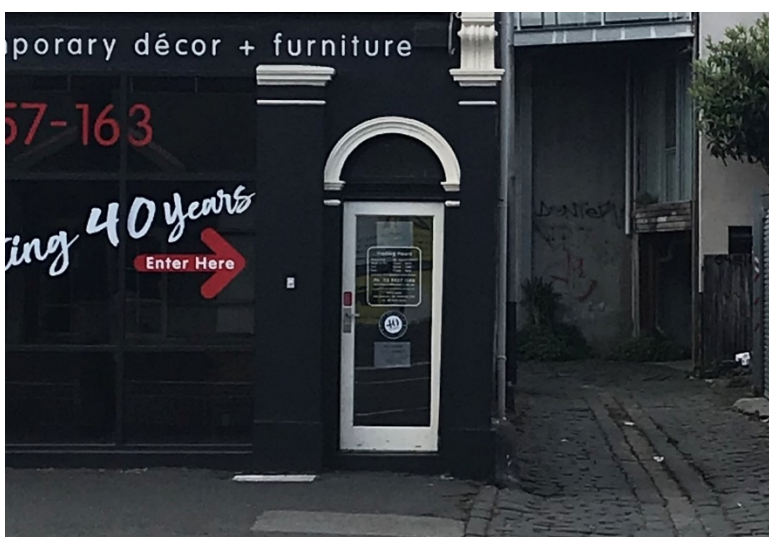
Figure 6: Detail view of the 'arched residential entry' at 163 Montague Street. The door is incorrectly described in the citation as original and timber panelled. This is not the case. Source: Trethowan Architecture, 2020.
