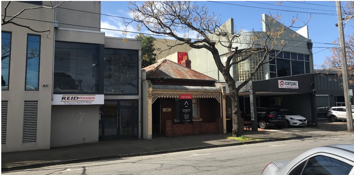
Figure 14: The house at 34 Boundary Street dates form c1900. Source: Trethowan Architecture, 2020.
