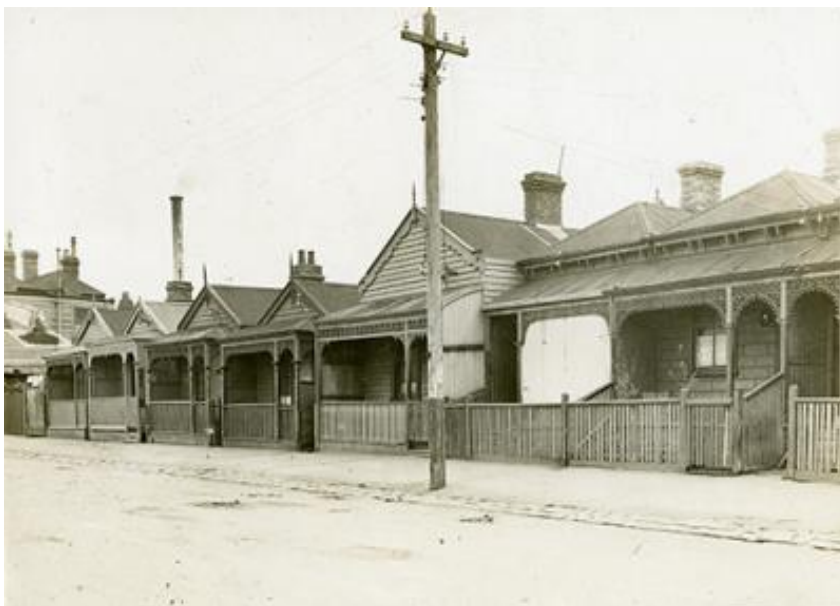
Figure 7: Gladstone Street looking west to Boundary Street c1930s. Source: Port Phillip Heritage Collection.
