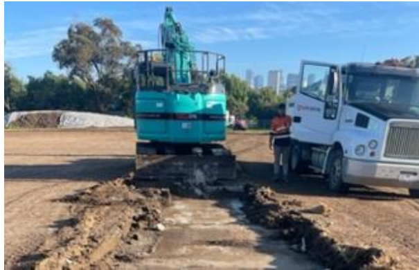
Works at Lagoon Reserve sports field.
