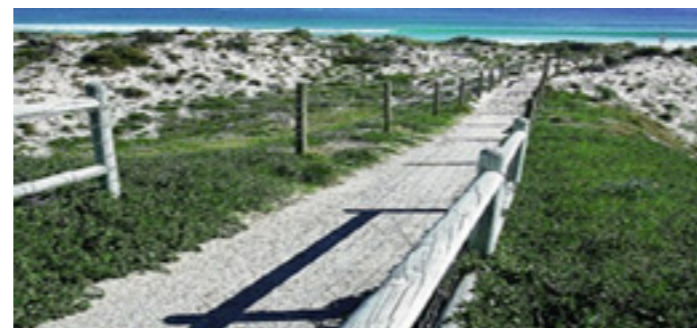
Example of coastal 'ring-lock and timber post' type fencing.
