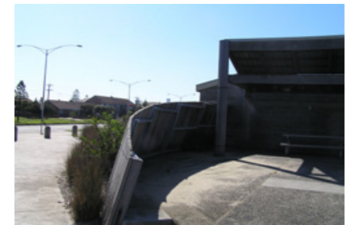
Curved, sloping timber wall will be used to unite Sandridge Pavillion (above) with the upgraded LSV frontage (Refer Appendix 2)
