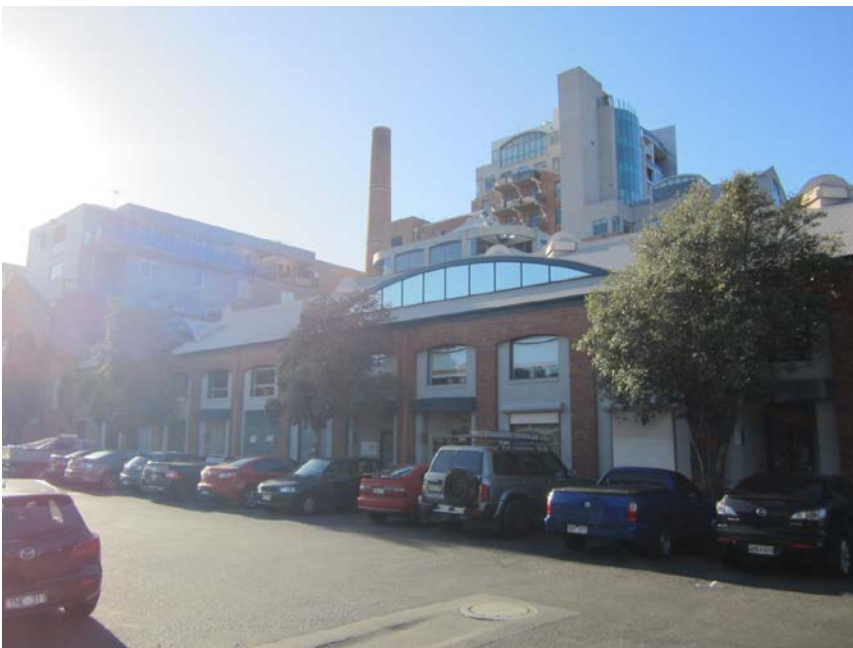
Figure 6 11 Beach Street showing elevation to Dow Street, looking east. This former single-storey warehouse building has been converted to a commercial use.
