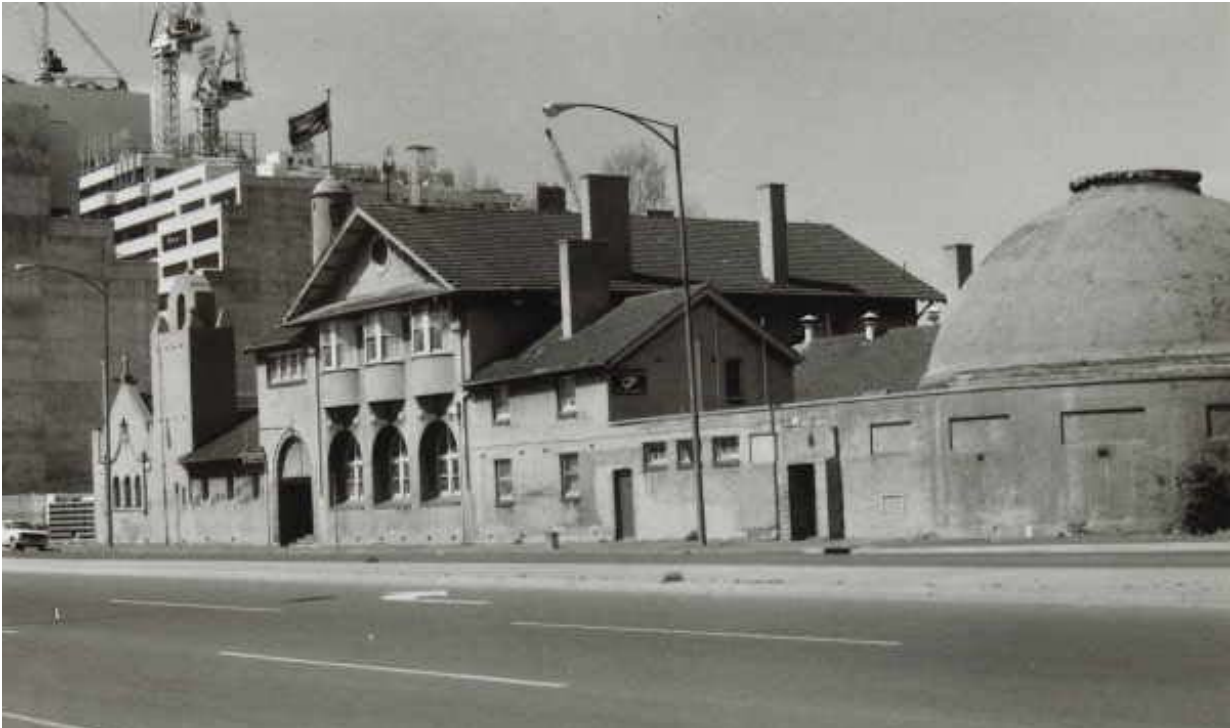
Figure 2 The former Anglican Missions to Seamen, now the Mission to Seafarers (1917), Flinders Street extension, Docklands, photographed in 1981. Source: John T Collins collection, State Library of Victoria.
