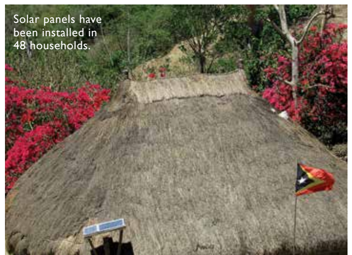
Installing the solar equipment.
