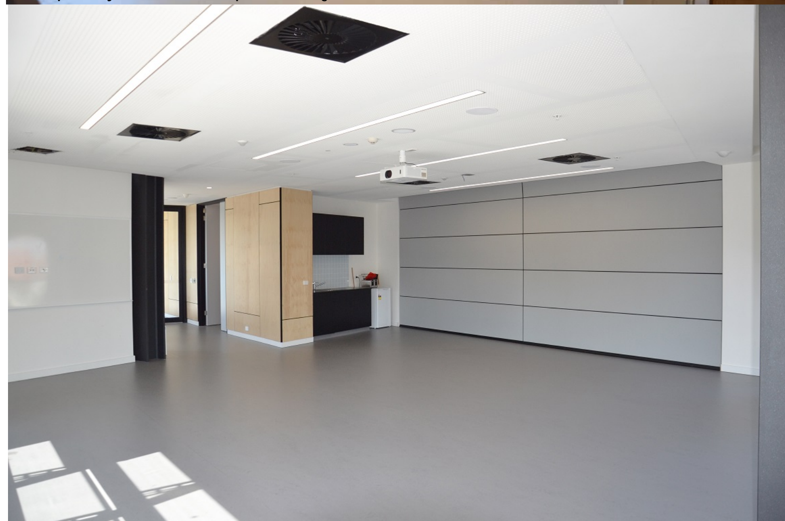
This multi-purpose can be divided into two separate spaces by an electric sound proof dividing wall.
