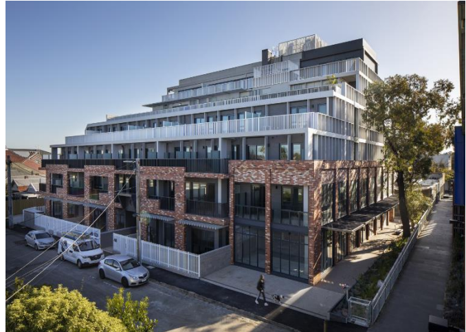
Marlborough Street community housing, Balaclava (Source: HousingFirst)
