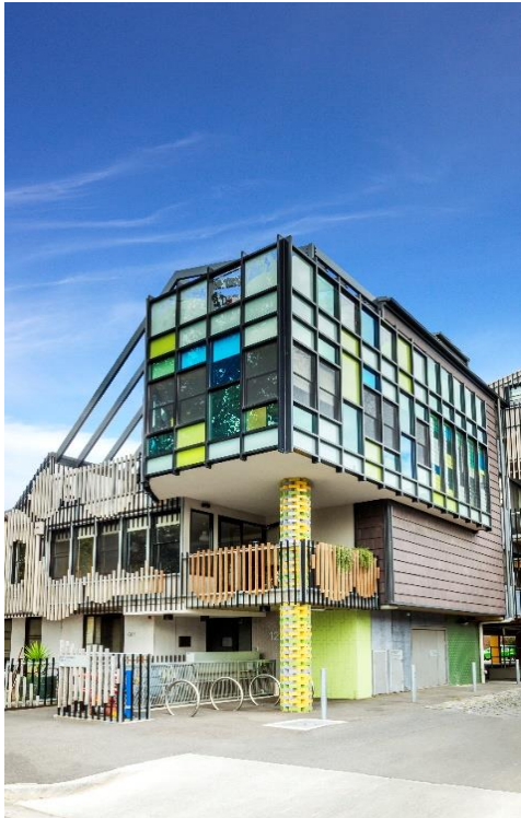
Kyme Place community housing, Port Melbourne (Source: City of Port Phillip)
