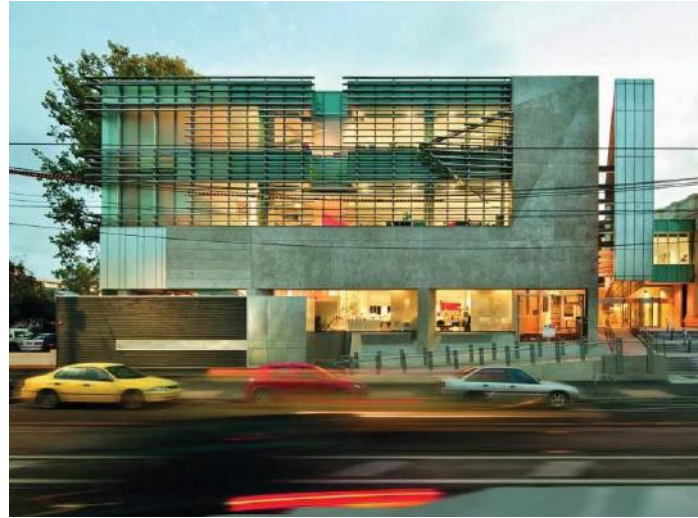
St.Kilda Town Hall Extension, Finalist for Best Non Residential Development, 2010 City of Port Phillip Design and Development Awards.
