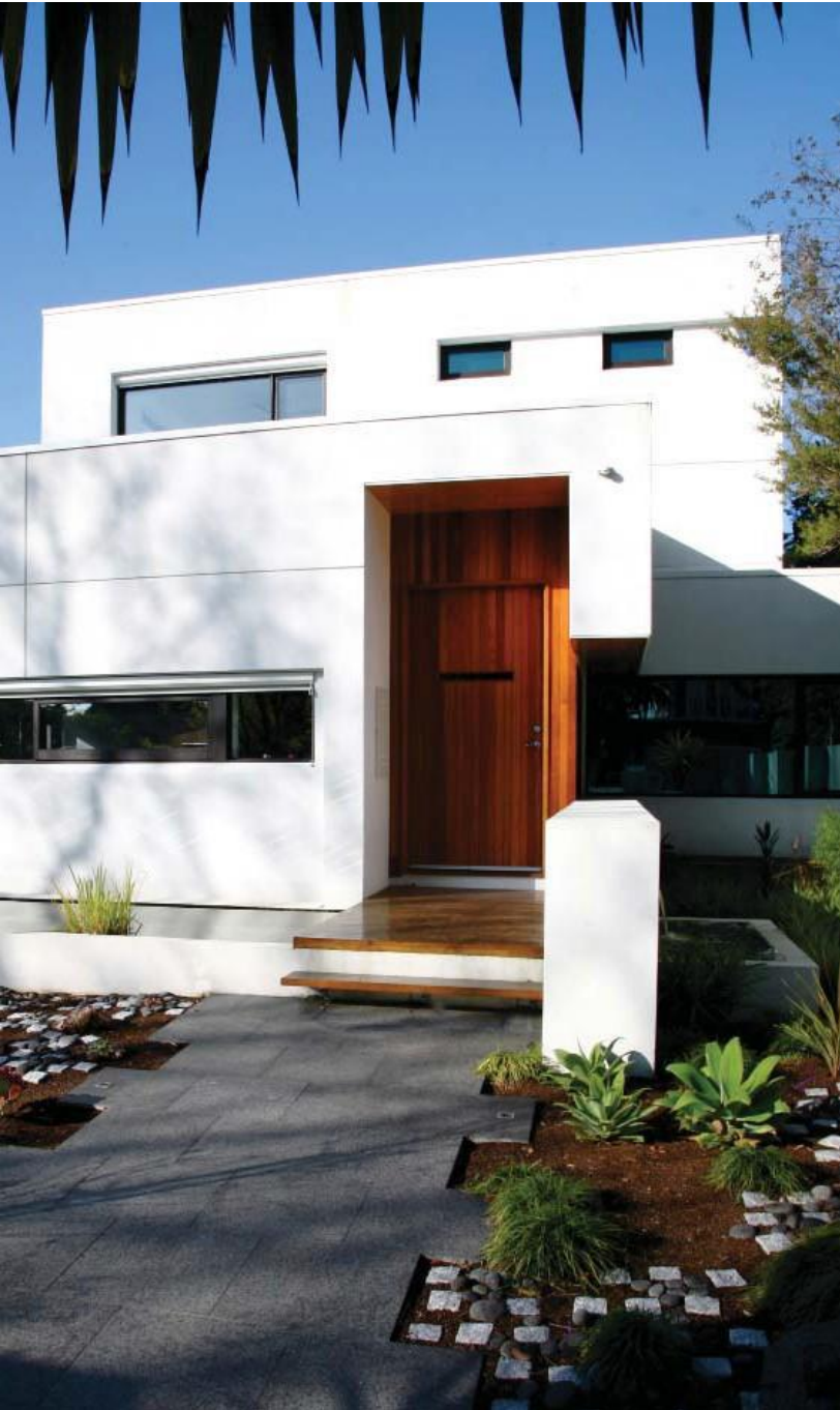
New Residence, Elwood.
