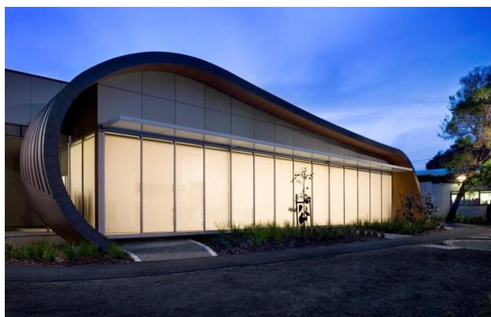
Betty Day Community Centre Architects: K20 Architecture
