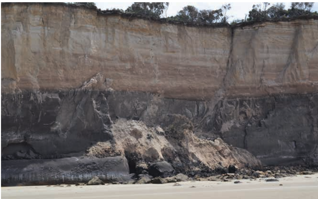
Coastal cliff erosion at Demon's Bluff, near Anglesea Geoff Wescott
