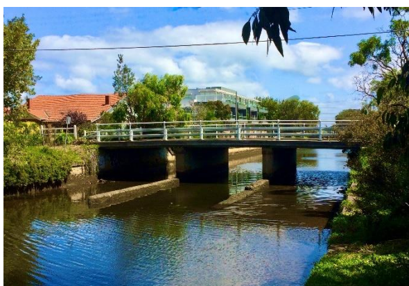
Broadway Bridge over Elwood Canal, Elwood.
