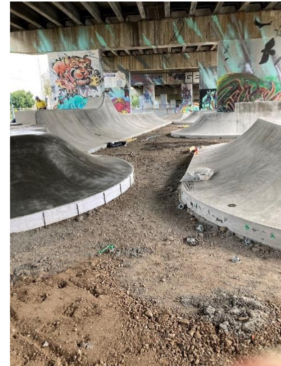
Port Melbourne Skate Park Construction Phase 1 works underway
