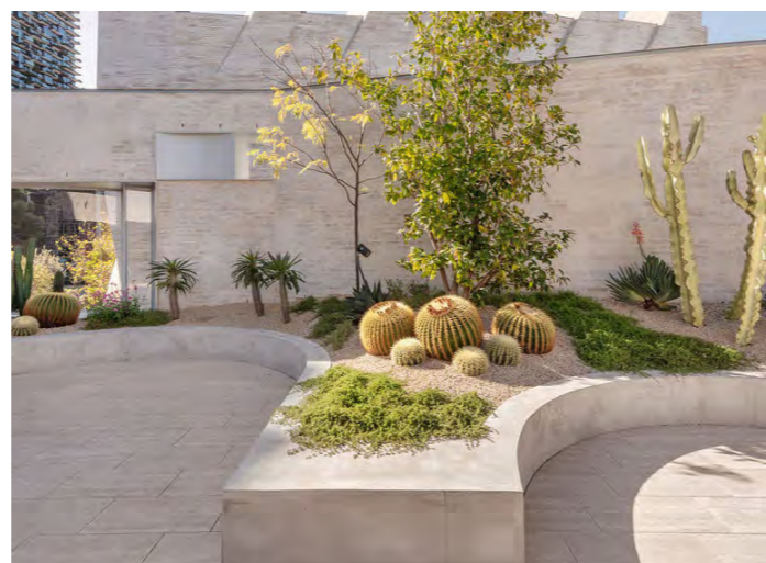
Curved concrete walls forming raised planters
