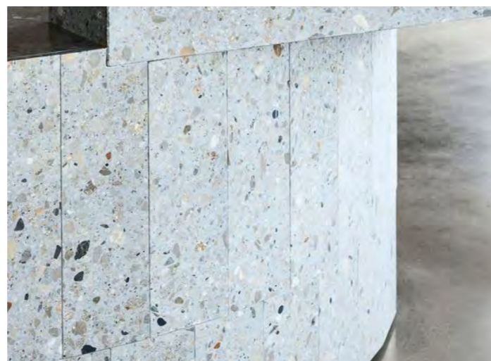
Exposed aggregate faceted concrete walls
