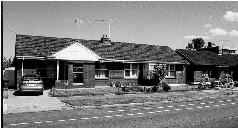
The dwelling to the left of the pair has an HCV porch and aluminium windows. That to the right has its original timber double hung windows and porch (now built in).
