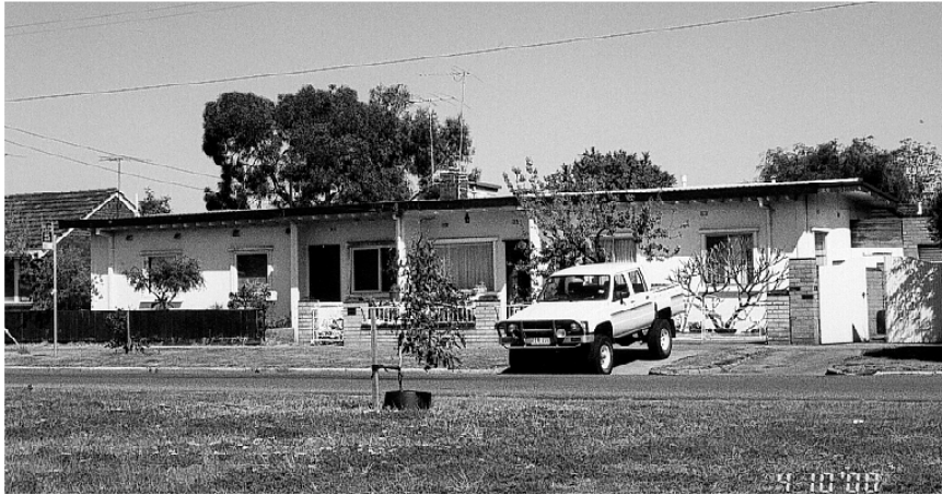
The first experimental dwellings using the TW Fowler system of concrete prefabrication, 324-326 Howe Parade, Fishermans Bend.
