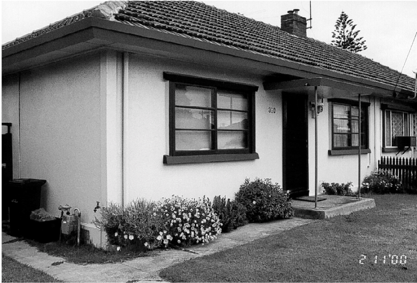
The original details of a concrete dwelling. Note the splayed eaves verge and splayed gutter, the eaves boxing, the partially concealed downpipe and the sliding timber windows with horizontal glazing bars set directly in the projecting concrete architrave in which the tracks are located.
