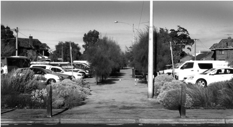
The two, two storey pairs of dwellings at the corners of Dunstan Parade and Centre Avenue frame the vista of the street. The vista was originally intended to be closed by the community centre.
