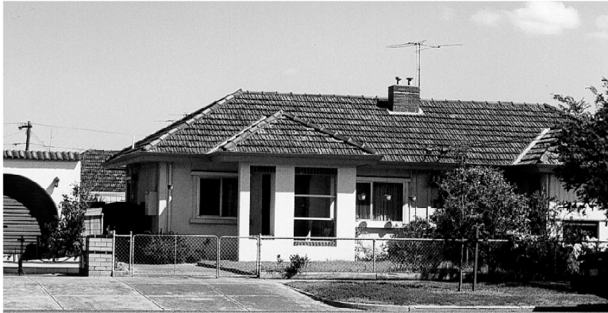
Later rendered brick porches on concrete dwellings.
