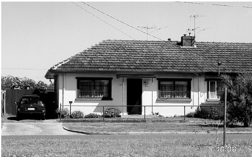
One of the most intact early concrete dwellings, 350 Howe Parade, Fishermans Bend. Note the splayed roof verge and gutter, the small concrete entry canopy carried on slender steel posts, the timber sliding sashes with horizontal glazing bars and the pipe and wire mesh fence
