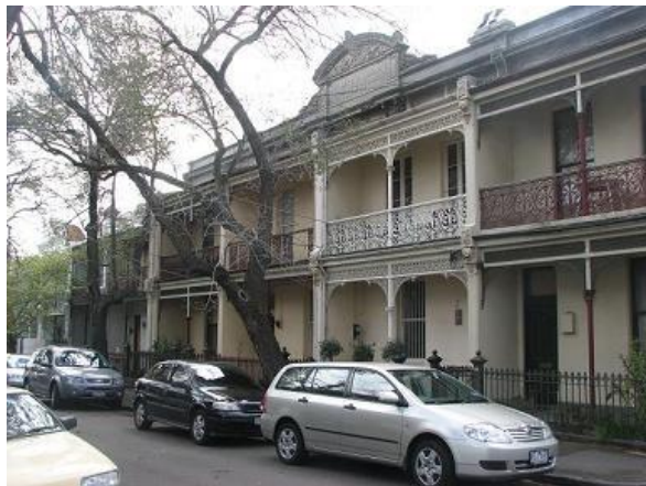
Figure 6.31-12 – Suo Marte Terrace (1885), a fine row of double-storey rendered terraced houses in Ward Street
