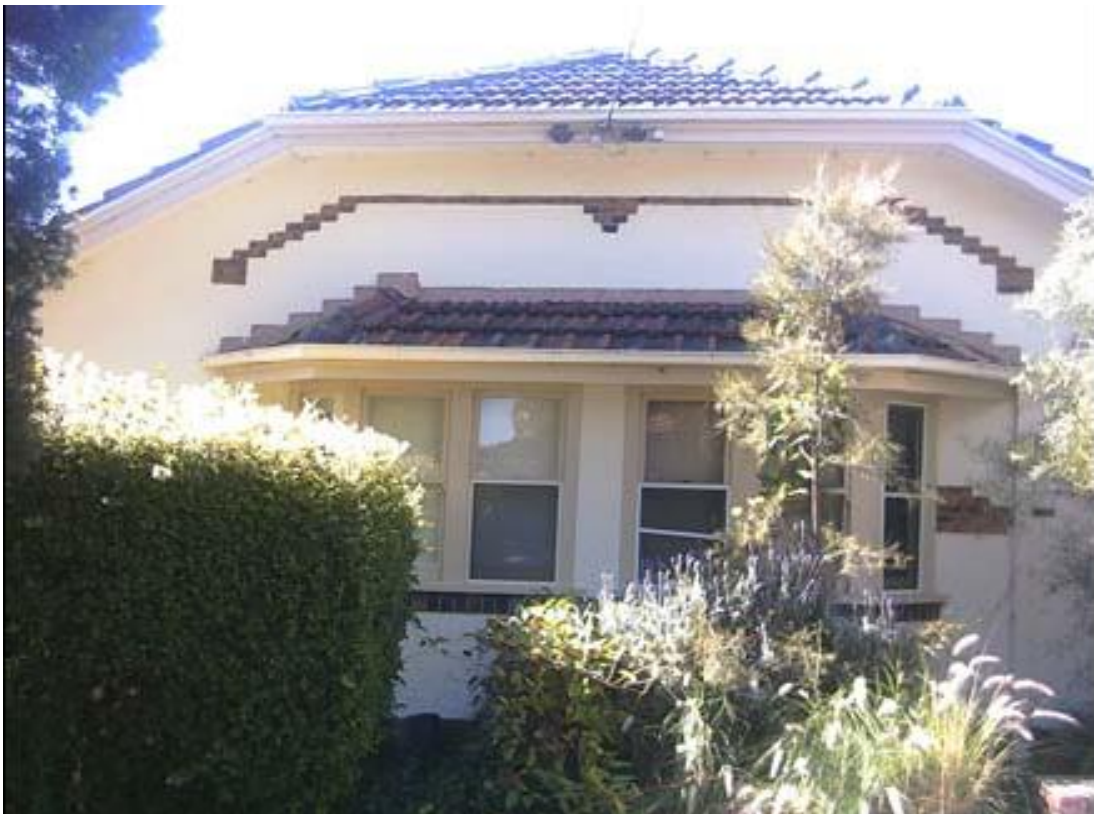
Figure 6.29-2 – Unique gambrel-roofed house at 4-6 McCrae Street, note: canted bay window across both dwellings
