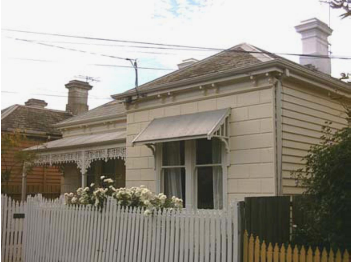
Figure 6.28–5 – Typical double-fronted timber villa, one of several in a row in Moore Street
