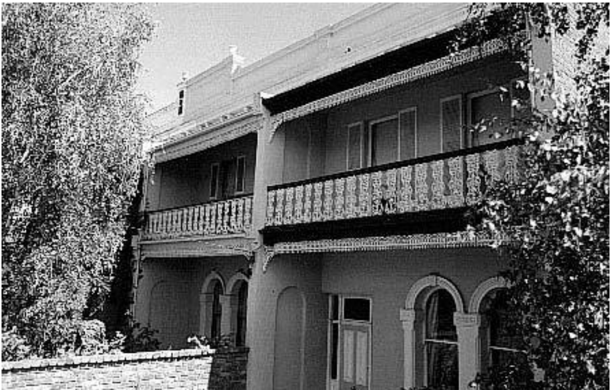
Figure 6.15-1 – The terrace at nos. 113-119 showing the Romanesque window heads that are a characteristic of the houses in this Area.
