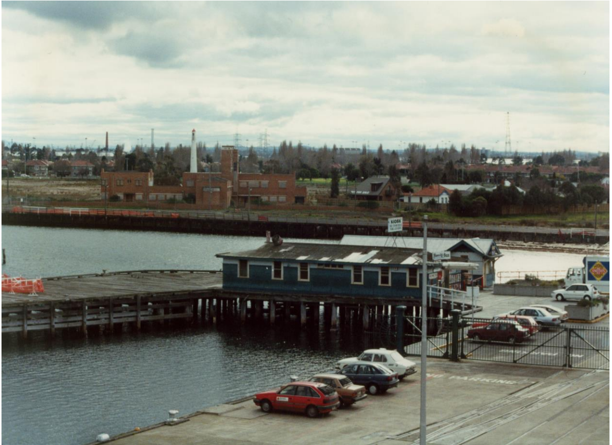
Figure 6.17-3 – Port Melbourne foreshore, including the Mission to Seamen Building and Swallow St
