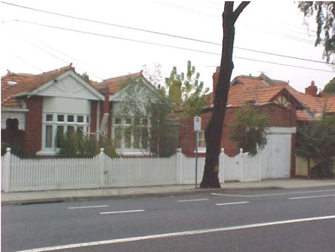
Figure 6.22-3 – 366 – 368 Inkerman Street, East St Kilda - note garage
