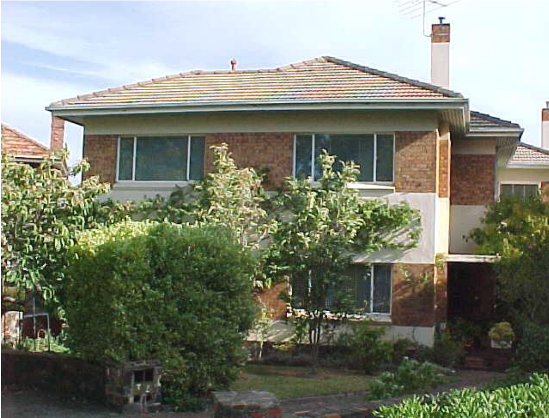
Figure 6.21-5 – Duplex, 4 – 5 Holroyd Court (1939)
