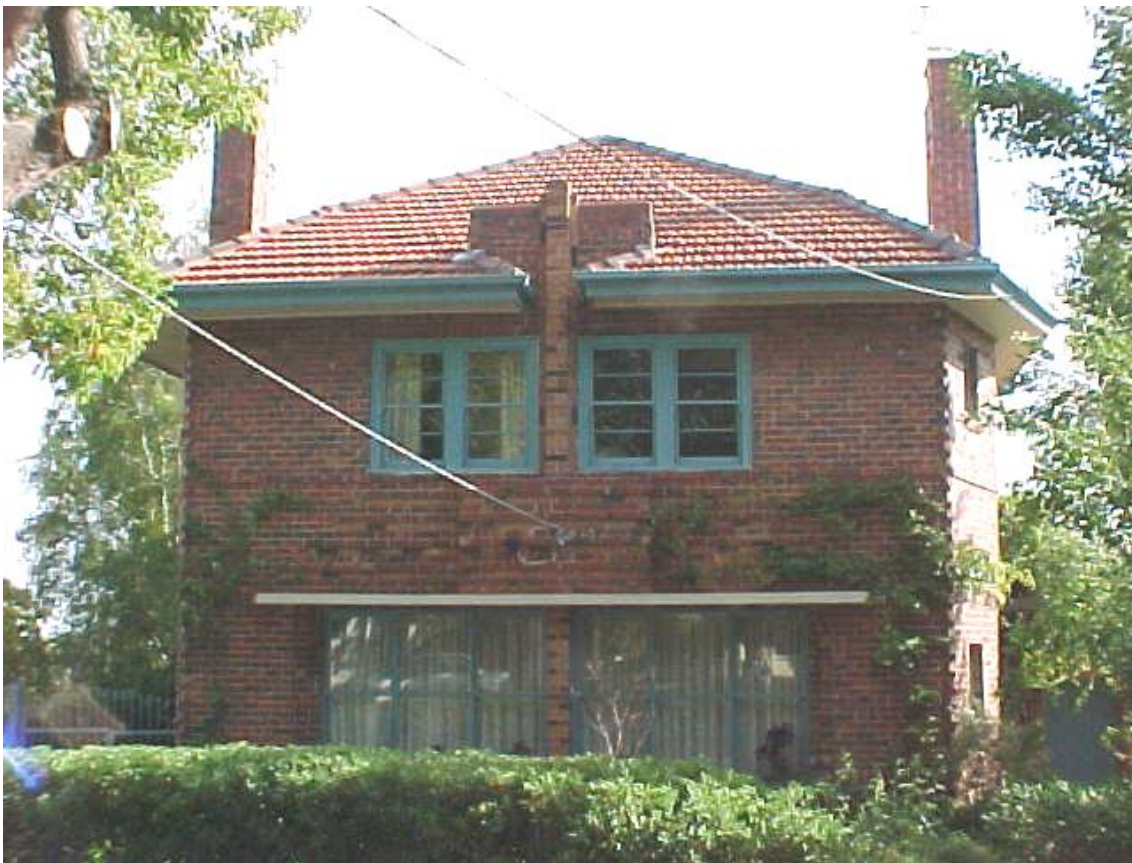
Figure 6.21-4 – Duplex, 2 – 3 Holroyd Court (1938)
