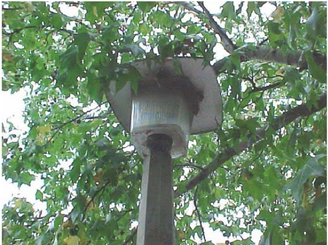
Figure 6.23-5 – Detail of 1920s concrete lamp
