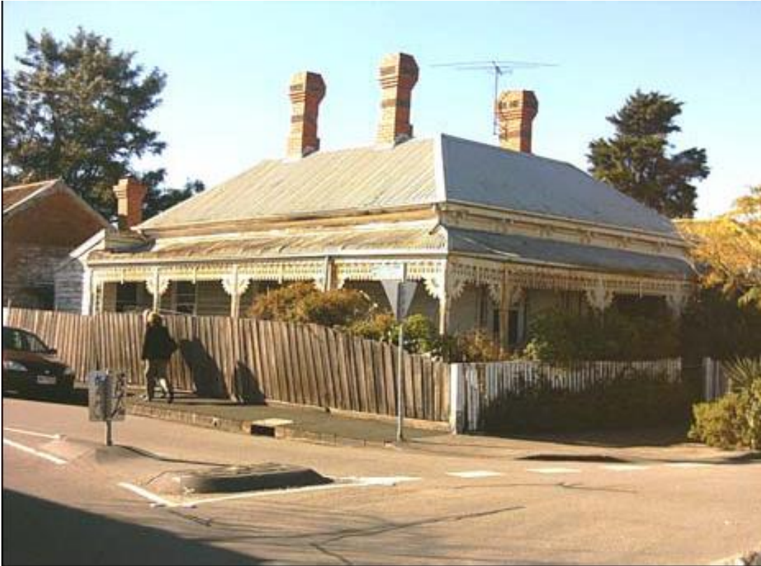
Figure 6.30-9 – 32 Nightingale Street; note return verandah and brick outbuilding.
