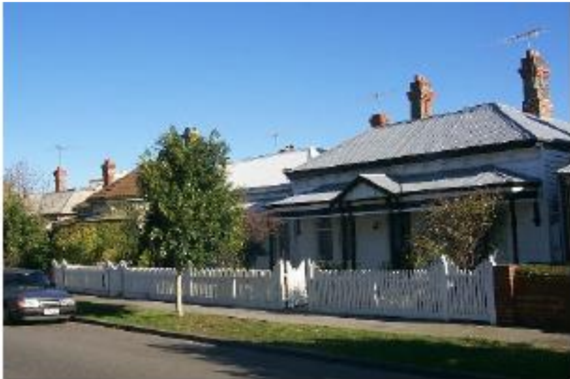
Figure 6.17-1 – Swallow Street, Port Melbourne
