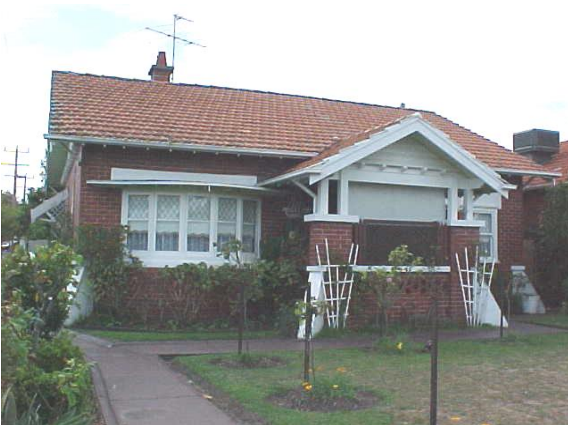
Figure 6.24-3 – Bungalow – 160 Alma Road (c.1925)
