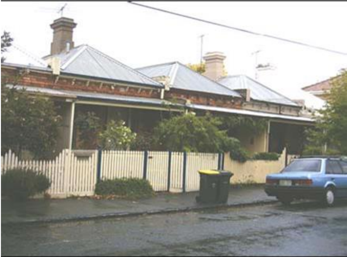
Figure 6.28-1 – Attached row of Victorian brick cottages at No 1-9 Moore Street
