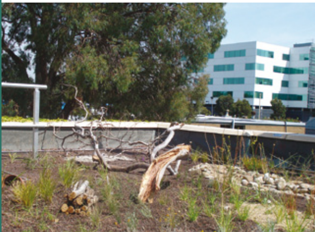
The Biodiversity Roof at The University of Melbourne's Burnley campus includes a range of substrate types and features to provide habitat opportunities for small wildlife. Note that this image shows the roof soon after construction. The plants will grow larger and less substrate will be exposed over time. Source: Peter Casamento
