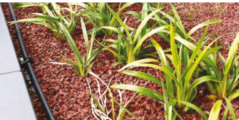
This green roof at the Peter Doherty Institute, Grattan Street, Parkville, functions as a grey water treatment system. Image: Eco Harvest
