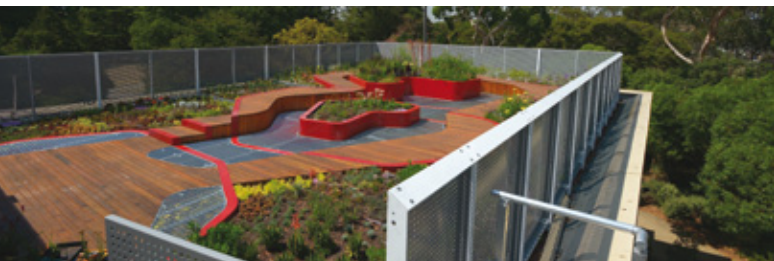
Perforated screens reduce wind flows on The University of Melbourne's demonstration green roof at Burnley campus
