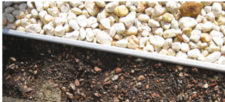
Edging can be used to separate different substrates on the roof
