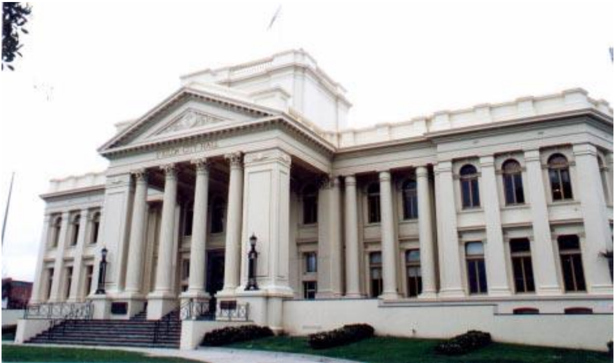
Figure 6.11-8 – The St. Kilda City Hall dominates the Carlisle Street/Brighton Road intersection and forms a group of public buildings with the St. Kilda School and the Holy Trinity Anglican church
