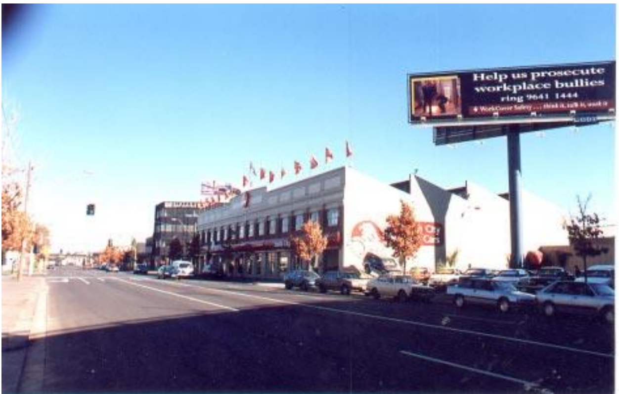
Figure 6.8–6 – Former General Motors Corporation headquarters, City Road, looking towards the railway overbridge.
