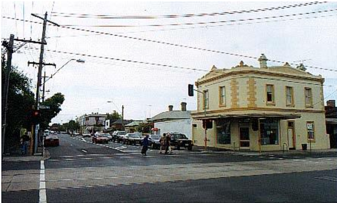
Figure 6.13-1 – Inkerman Street, south side, looking east from Chapel Street at a point of entry to the Area
