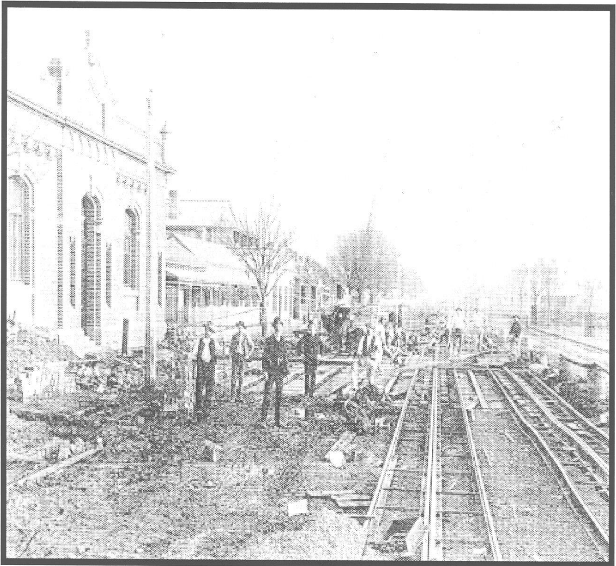
Figure 6.8-3 – City Road in 1890, showing the cable tramway being installed with the engine house at left. Notice the absence of development on the right hand side of City Road.
