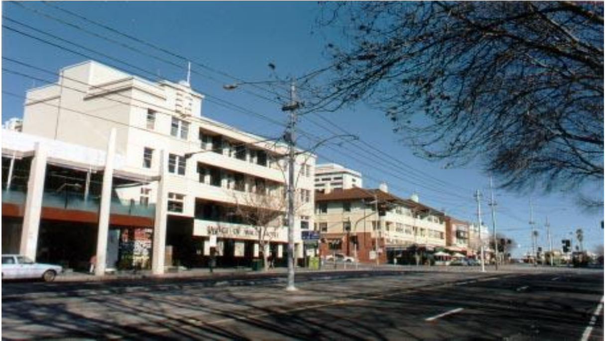
Figure 6.9–8 – Fitzroy Street, showing “The Prince of Wales” hotel, designed by R.H. McIntyre and built in 1937 with “Summerland Mansions”, designed by Christopher Cowper and built in 1920-21: both temples to St. Kilda’s role as a seaside resort.
