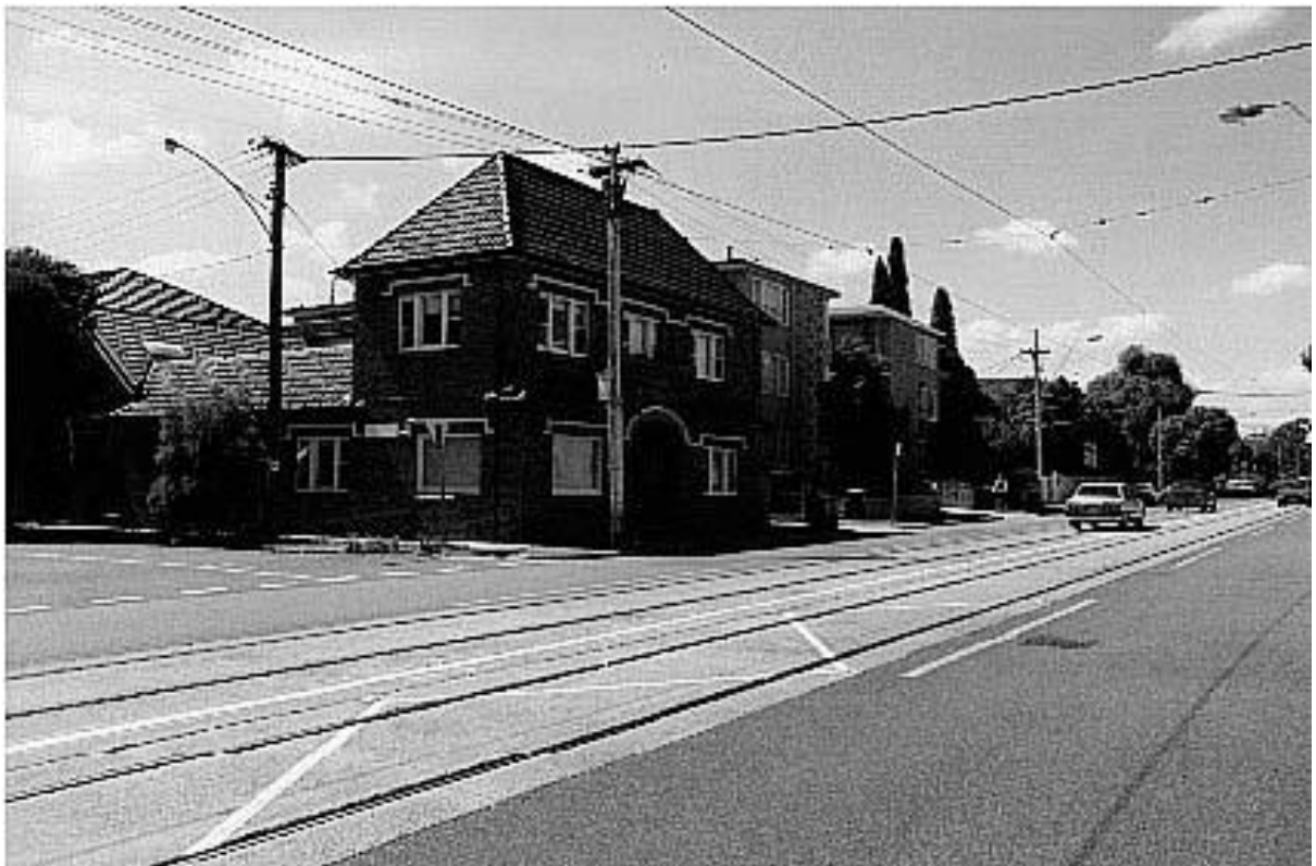
Figure 6.14-4 – The north side of Carlisle Street, looking east from the Kollel Beth Hatalmud Yehuda Fishman Institute which is diagonally opposite “Astolat”.
