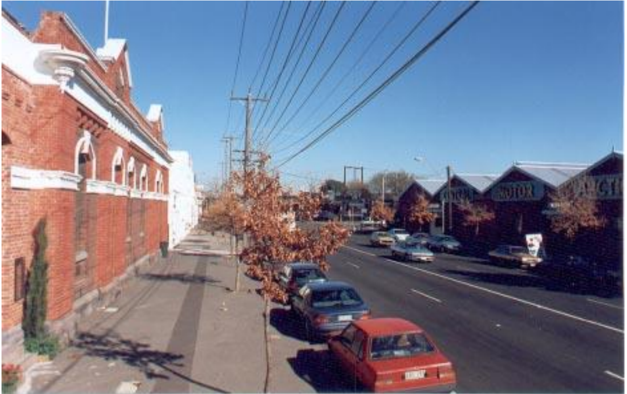
Figure 6.8–5 – City Road, with the former cable tramway engine house at left and the former Johns and Waygood factory at right.
