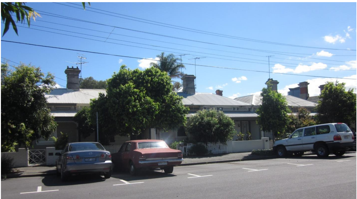
Figure 6.3–7 – Paired timber villas in Ross Street, north of Bridge Street with central rendered brick chimneys.
