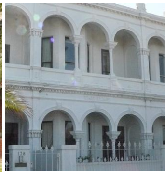
Figure 6.35–12 – Row of Double -storey terrace houses, Beaconsfield Parade
