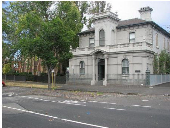
Figure 6.32-7 – Former doctor's townhouse (later RAIA offices) at 30 Howe Crescent, with polychrome church alongside
