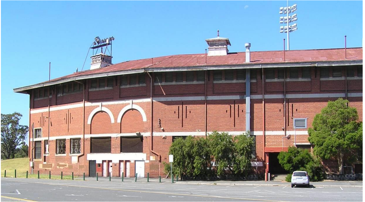
Figure 6.38-10 – The west elevation of the South Melbourne Grandstand, showing row of highlight windows beneath the eaves.
