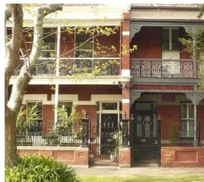
Figure 6.35–11 – Set of Double-store terrace houses, Mary Street
