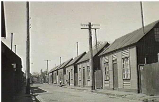
Figure 6.31-3 – Robert Patterson’s two-roomed prefabricated iron cottages in Patterson Place, still intact in a photograph taken in 1933
