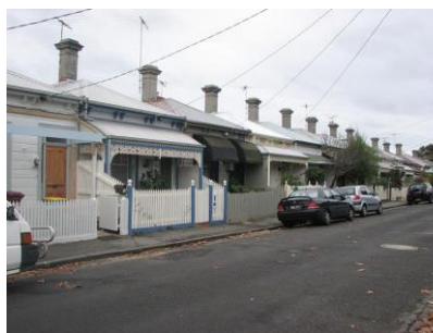
Figure 6.35-8 – Row of single-fronted Victorian timber cottages, Erskine Street
