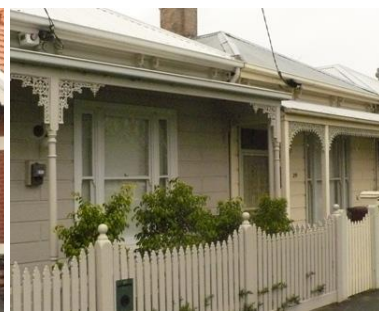
Figure 6.35–18 – Row of Victorian timber cottages, Middle Park
