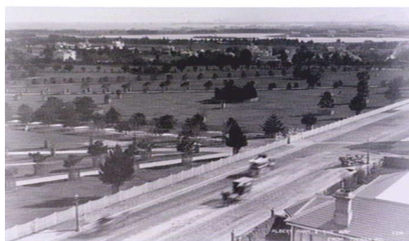
Figure 6.37-2 – Aerial photograph of Albert Park, 1900
