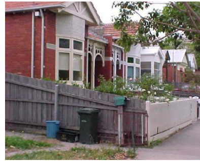
Figure 6.35-20 – Edwardian red brick villas in Inkerman Street, St Kilda East
