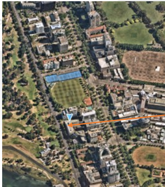
Figure 5 – Aerial of surrounding area 7
