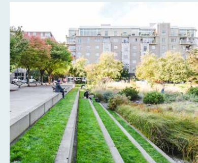
Designing public spaces to reduce the impacts of flooding - parks, sports fields and roads that retain water during severe storms.
