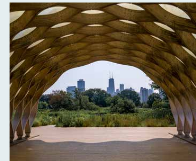
Designing flexible pavilion spaces that offer shelter from sun or rain, and can be programmed for community events such as performances, fitness classes and social gatherings.
