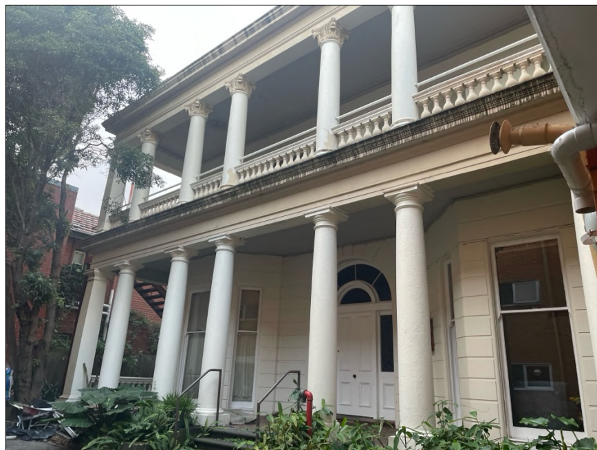
Figure 6 View of the facade, with original columns and balustrade to the upper level verandah.
