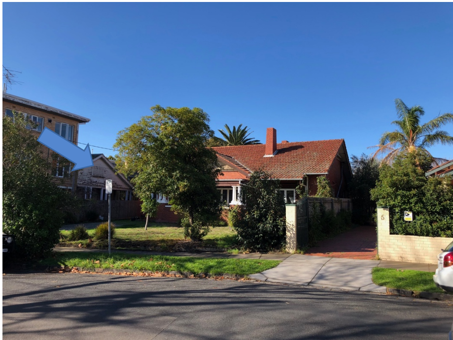
Figure 8: An early house in the street is extant behind a block of 1960s flats at 1 Tiuna Grove (indicated with arrow).
