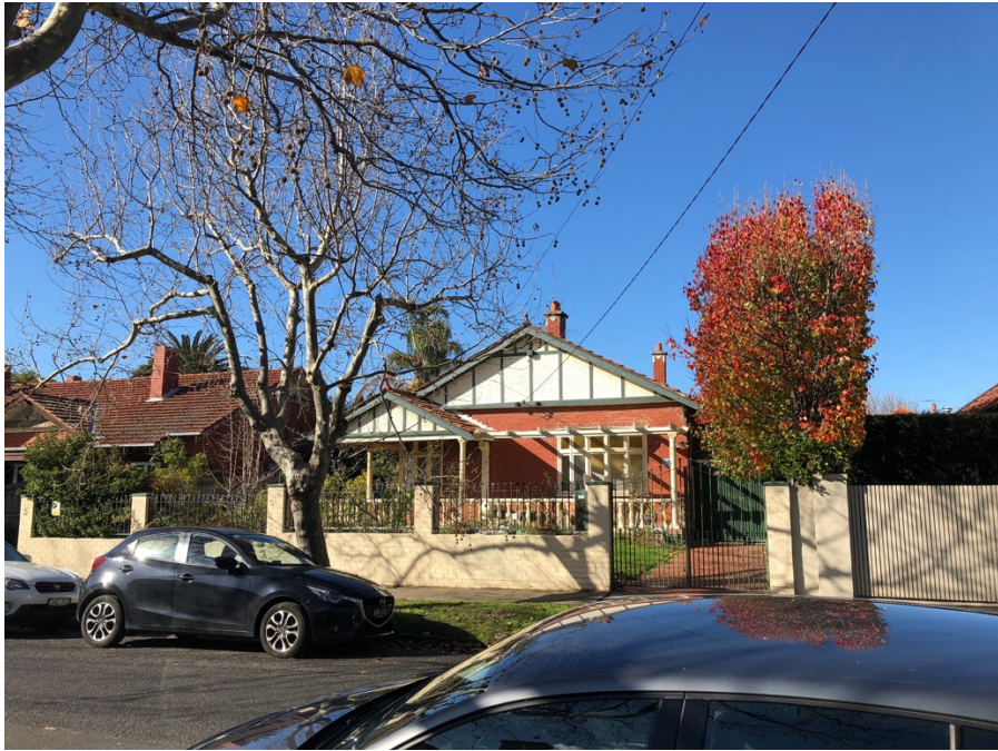
Figure 5: Bungalow at 5 Tiuna Grove proposed for an interim heritage overlay.
