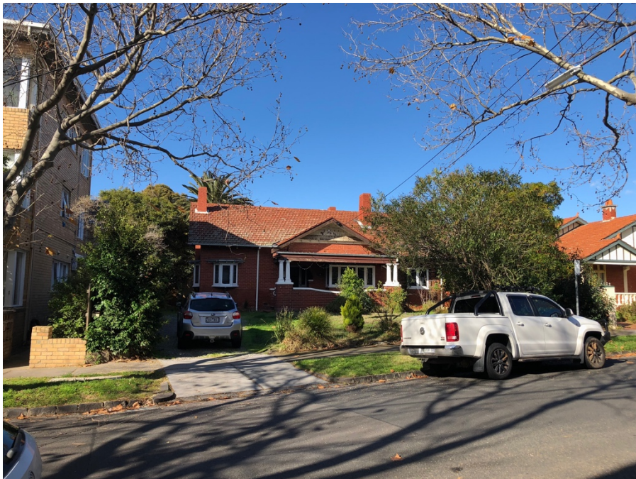
Figure 4: Bungalow at 3 Tiuna Grove proposed for an interim heritage overlay.
