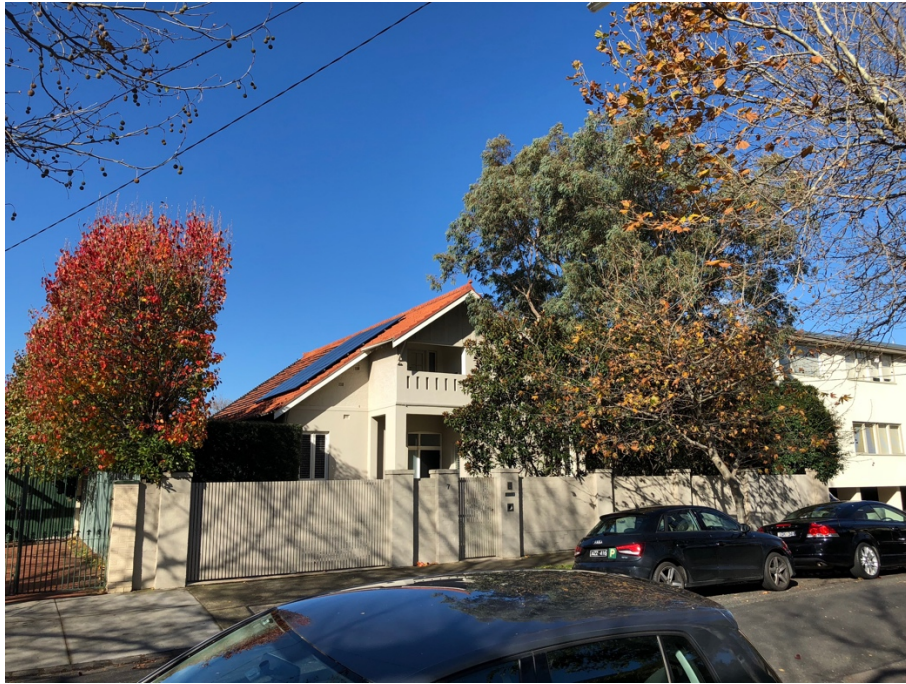
Figure 7: Bungalow at 7 Tiuna Grove proposed for an interim heritage overlay.
