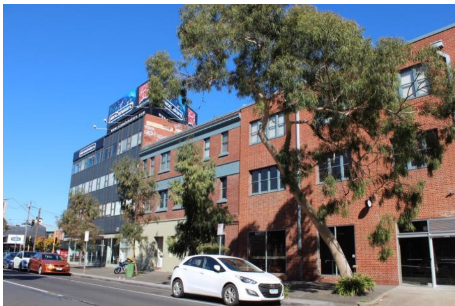
Figure 2 - 1960s office on corner of Cecil Street, c1910 general store and c1920 machine shop on right.
