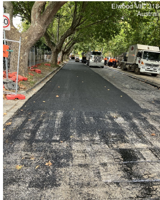
Images left: Broadway Street road upgrade, Elwood
