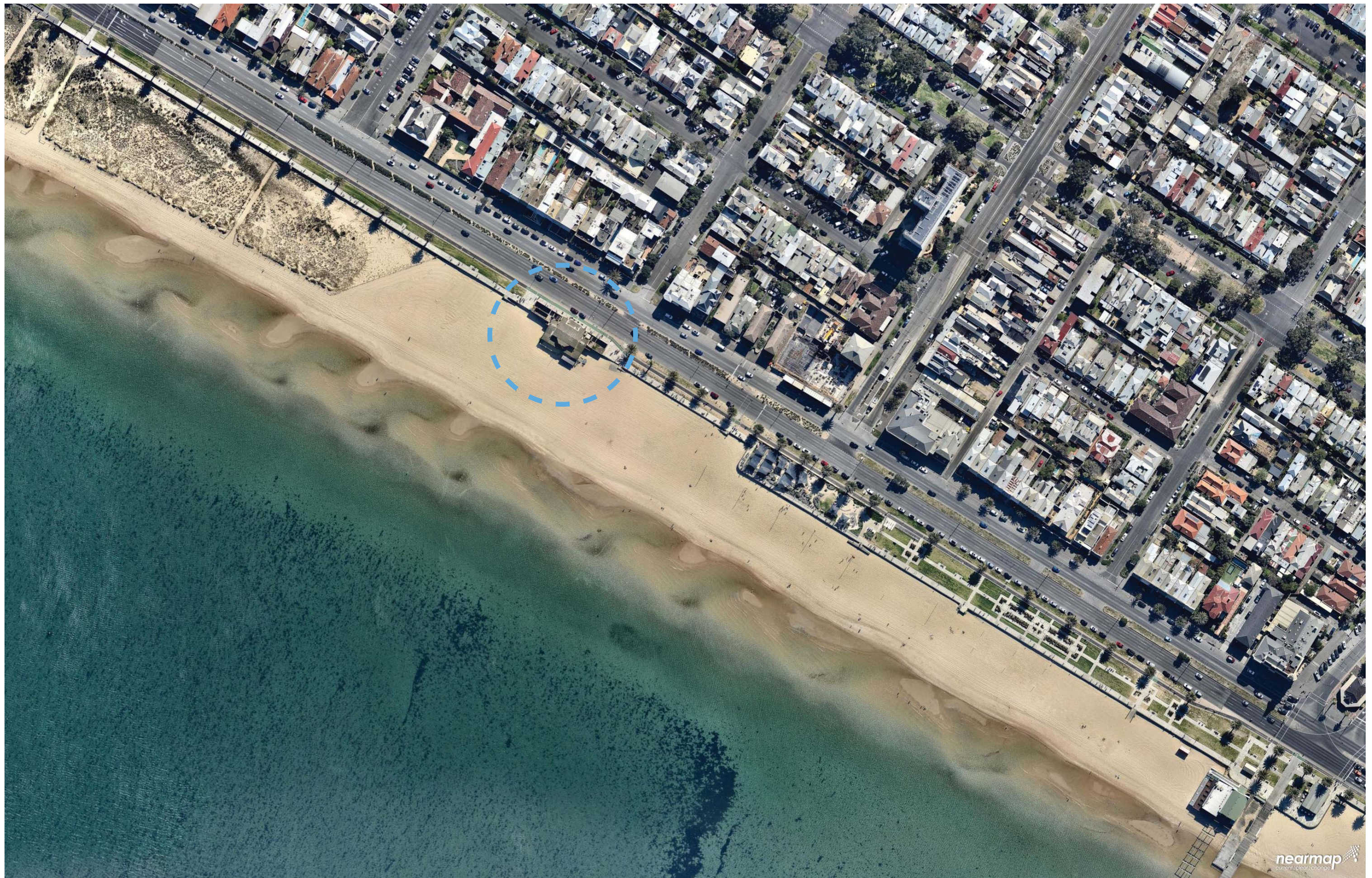
AERIAL VIEW OF THE EXISTING SOUTH MELBOURNE LIFE SAVING CLUB BUILDING
