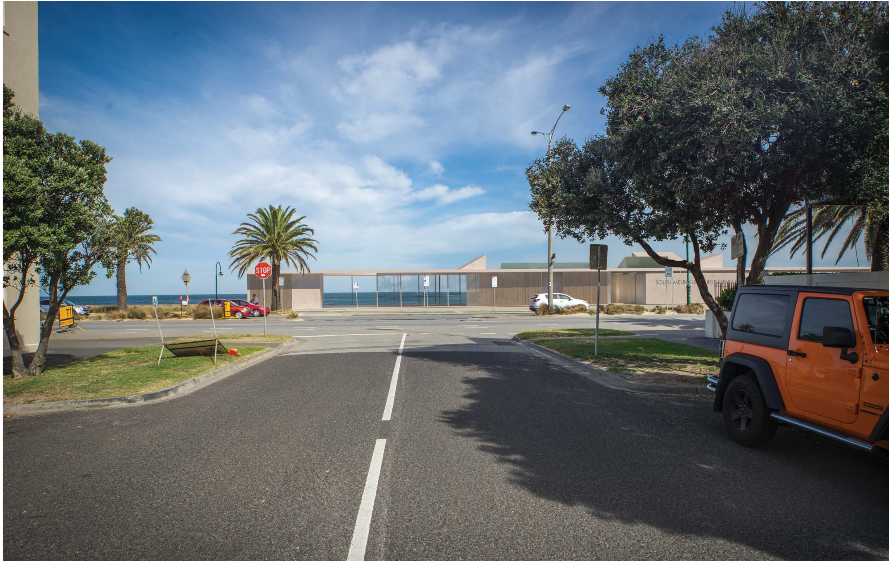
CONCEPT DESIGN - ARTISTIC IMPRESSION OF NEW BUILDING FROM WITHERS ST - SLIDING SCREEN OPEN
