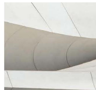
CD:02 Concrete Look Finish
