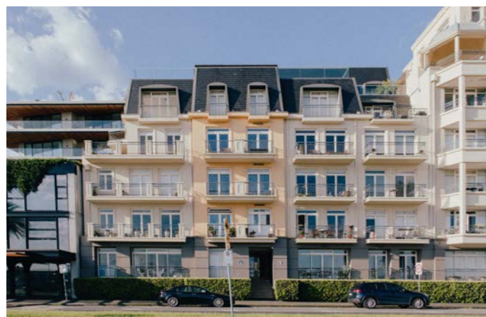
Residential Character of Beach Street
