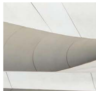
CD:02 Concrete Look Finish
