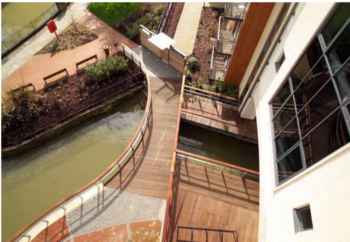
A flood proof building
