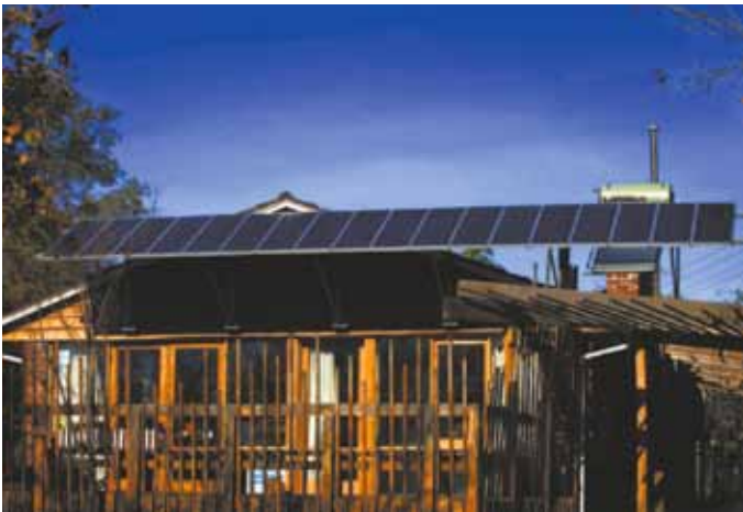
The EcoCentre, St Kilda uses well positioned solar panels to provide summer 'eaves'
