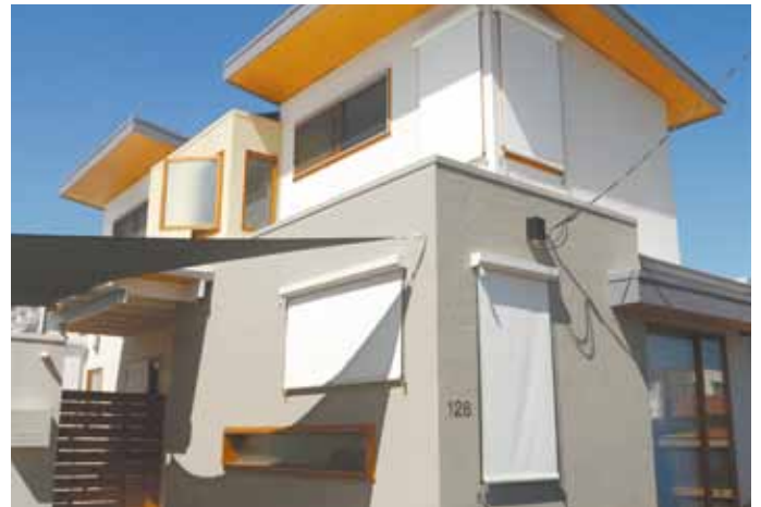
This house in Ross Street, Port Melbourne incorporates wide eaves and external blinds to reduce summer heat indoors
