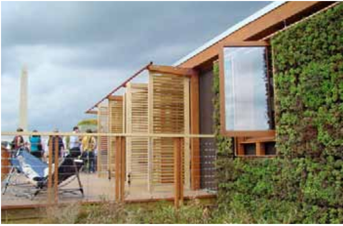
Eaves, shutters and green walls aid temperature control and ventilation
