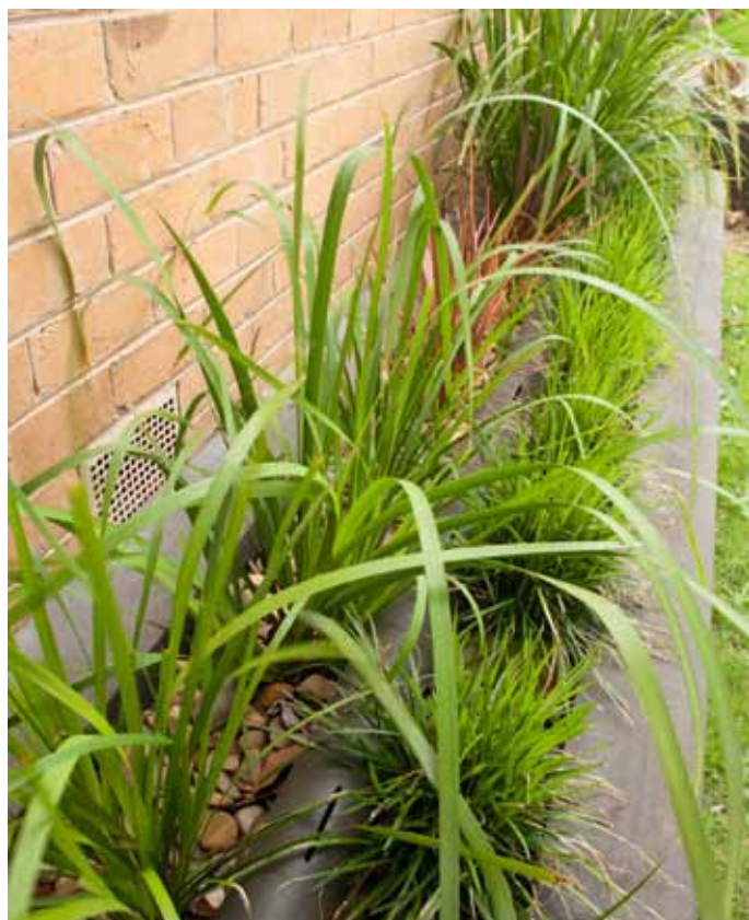
A raingarden channels and cleans stormwater, and helps to reduce stormwater runoff. Image: Courtesy Melbourne Water
