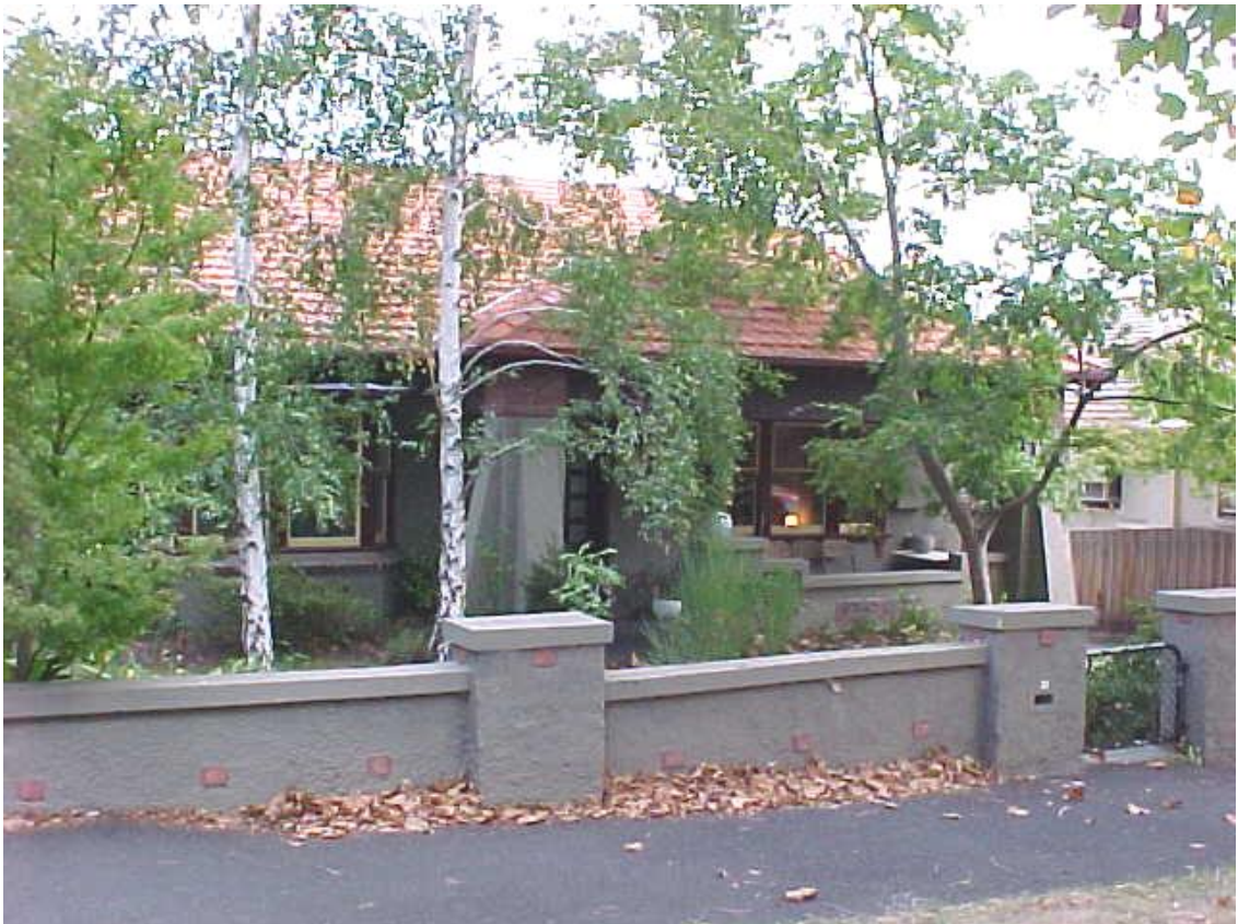
Figure 6.24-3 – Jacka's house at No. 23 Murchison Street (1924)
