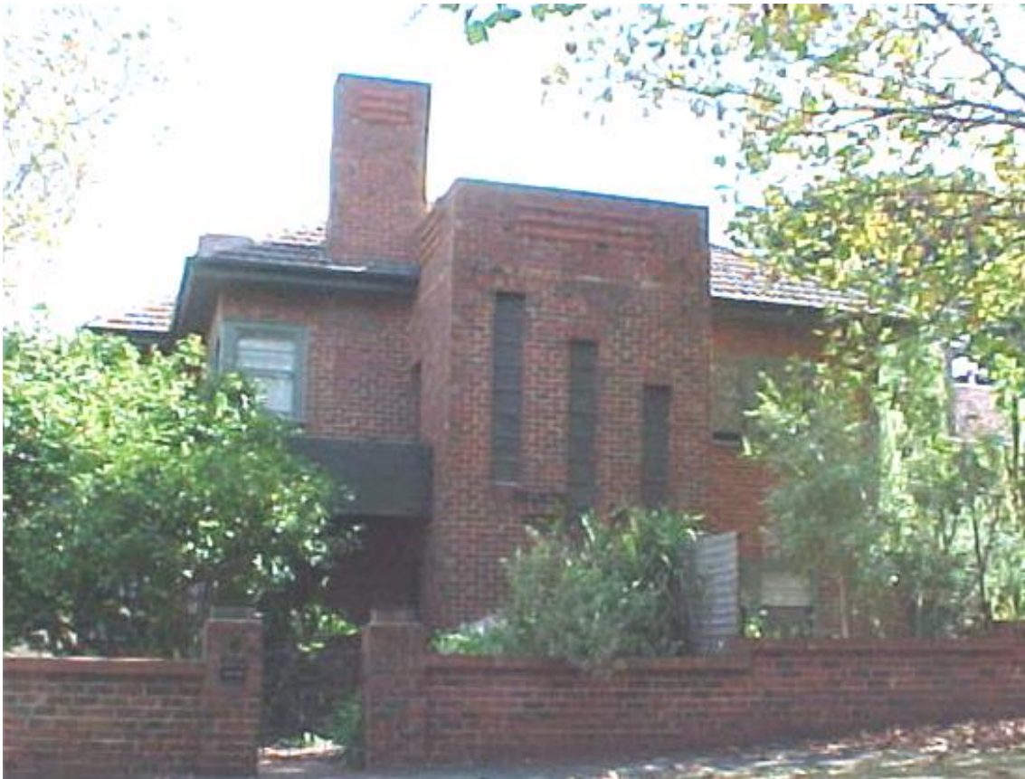
Figure 6.24-4 – Flats, 18 Murchison Street (1938)
