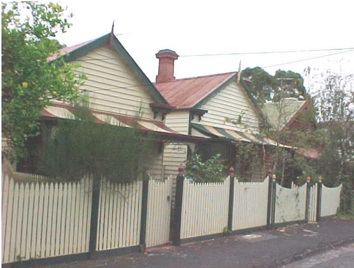
Figure 6.18-2 – Chusan Street, East St Kilda - looking north
