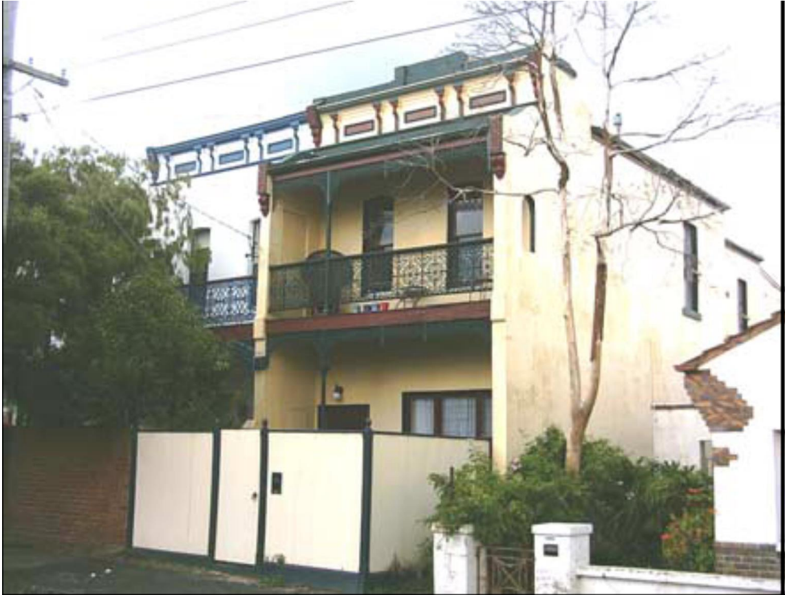
Figure 6.28–4 – Atypical pair of rendered Victorian double-storey terrace houses at 15-17 Byron Street
