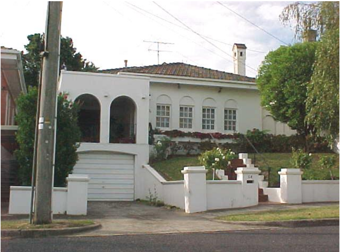
Figure 6.23-3 – House at 14 Mooltan Avenue (c.1928)
