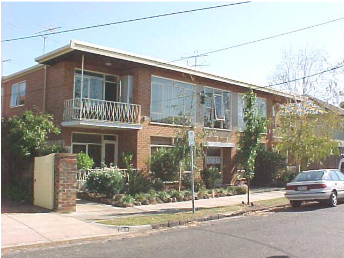
Figure 6.25-7 – Post-war flats at No. 22 Orange Grove (c.1966)
