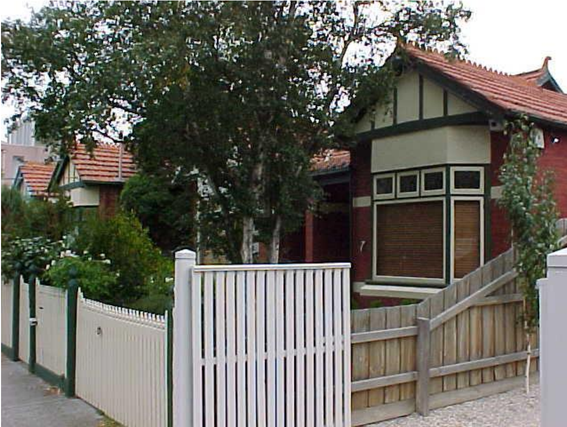
Figure 6.22-1 – Row of houses 1 – 7 Kalymna Grove, East St Kilda
