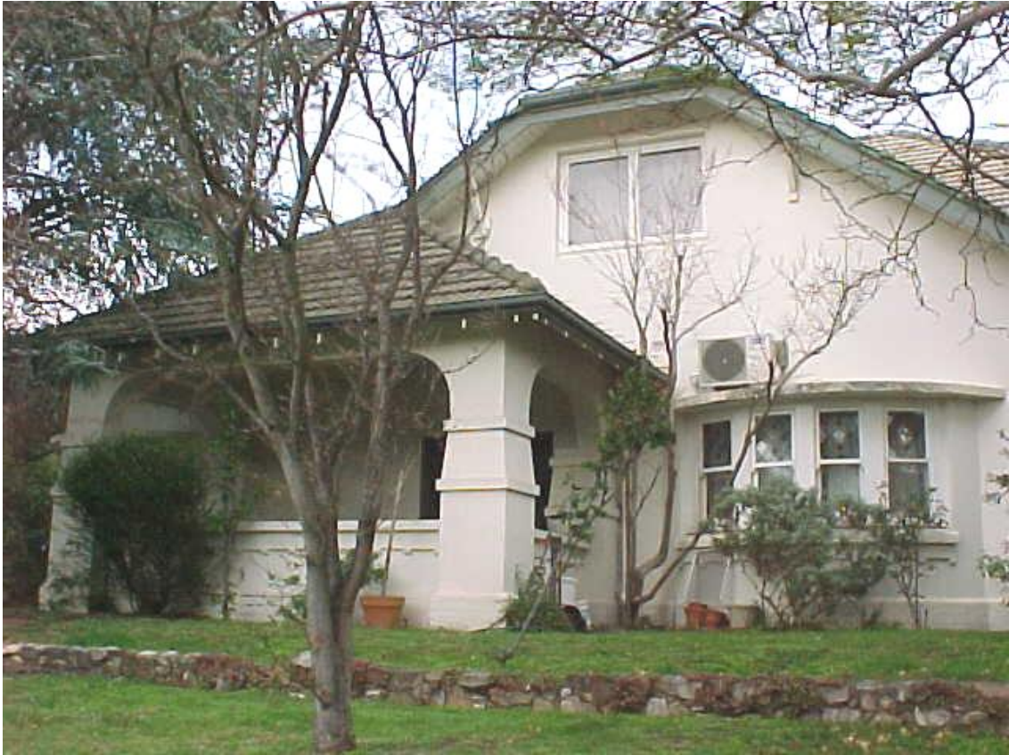
Figure 6.24-6 – Attic bungalow, 211 Alma Road, East St Kilda
