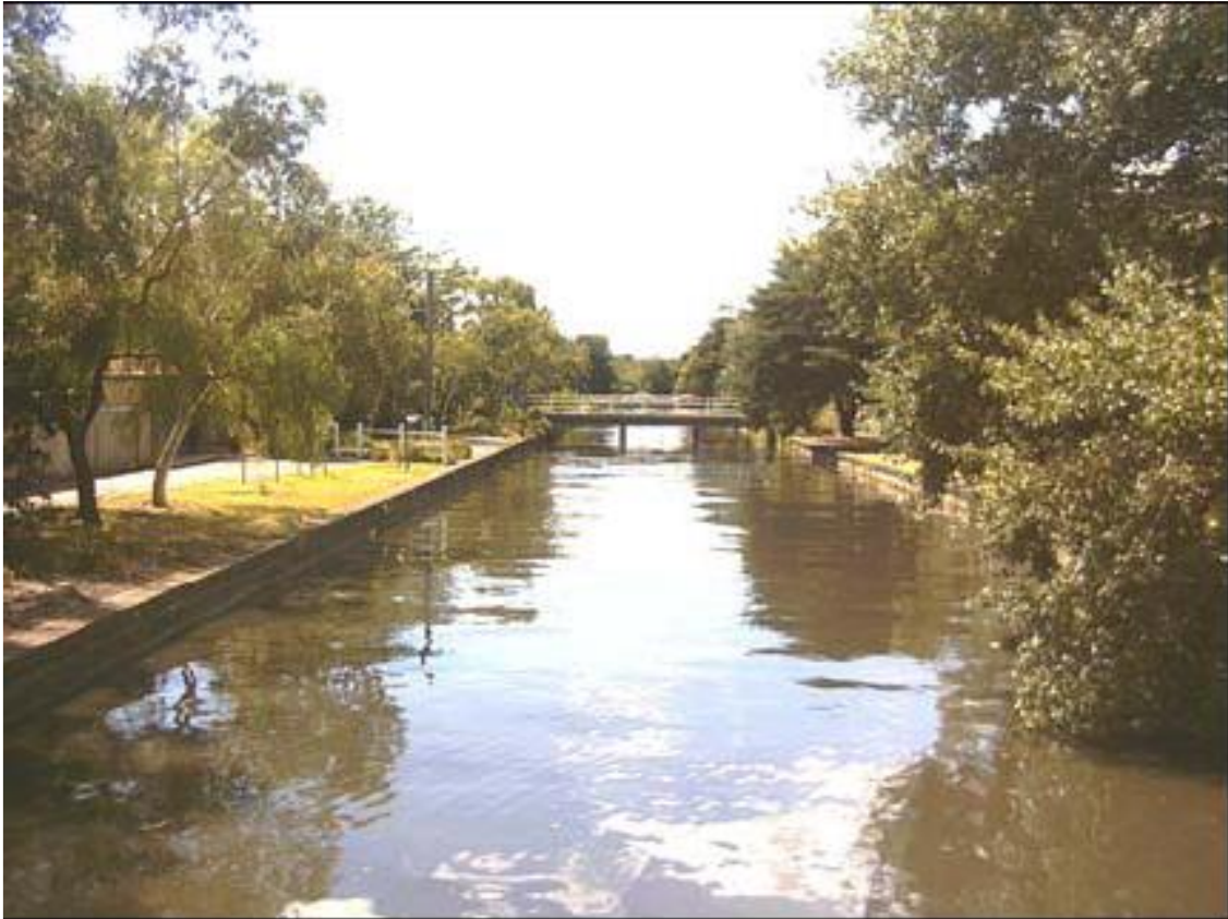
Figure 6.26–2 – General view of the Elwood Canal; photograph taken after flood rains (Feb 2005)
