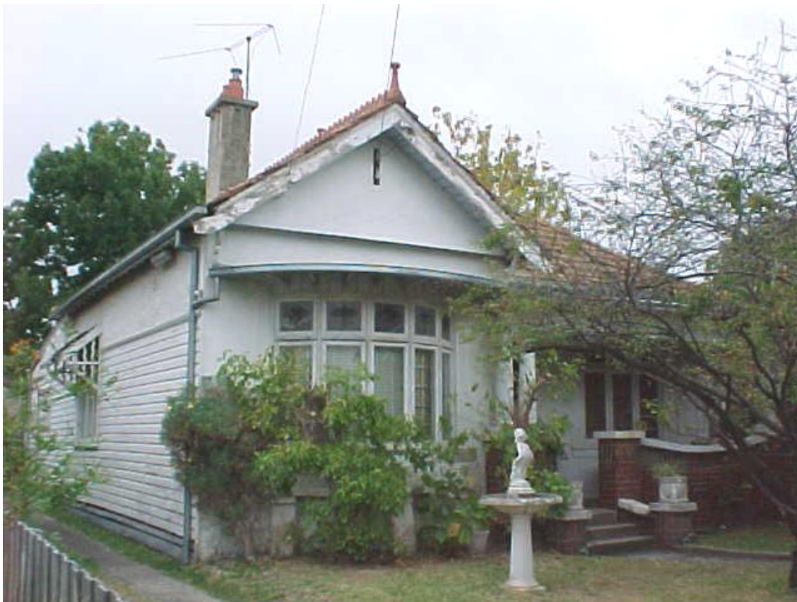
Figure 6.22-4 – Weatherboard House at No.6 Kalymna Grove, East St Kilda
