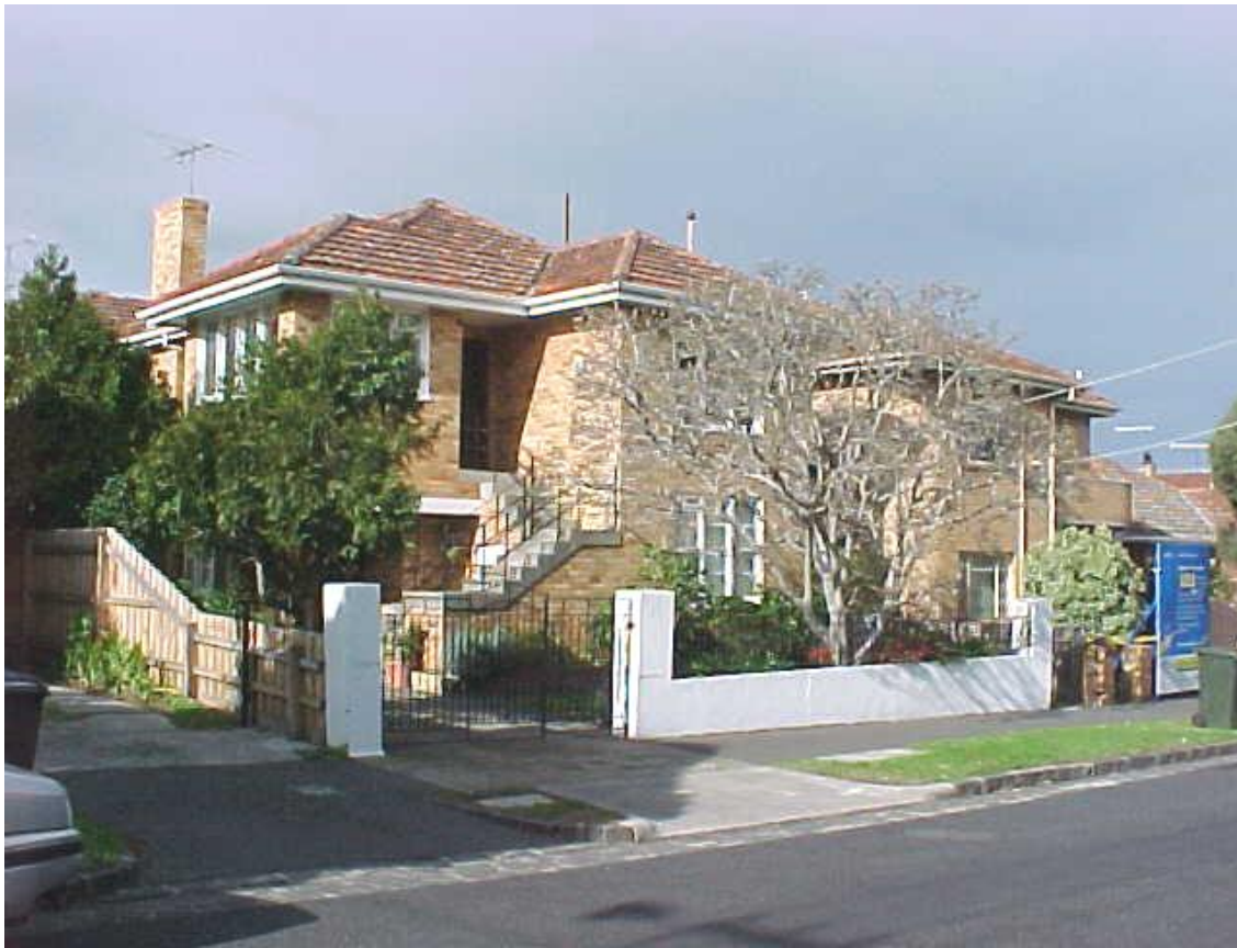
Figure 6.20–8 – Double storey flats at Nos 4 and 6 Hammerdale Avenue, East St Kilda
