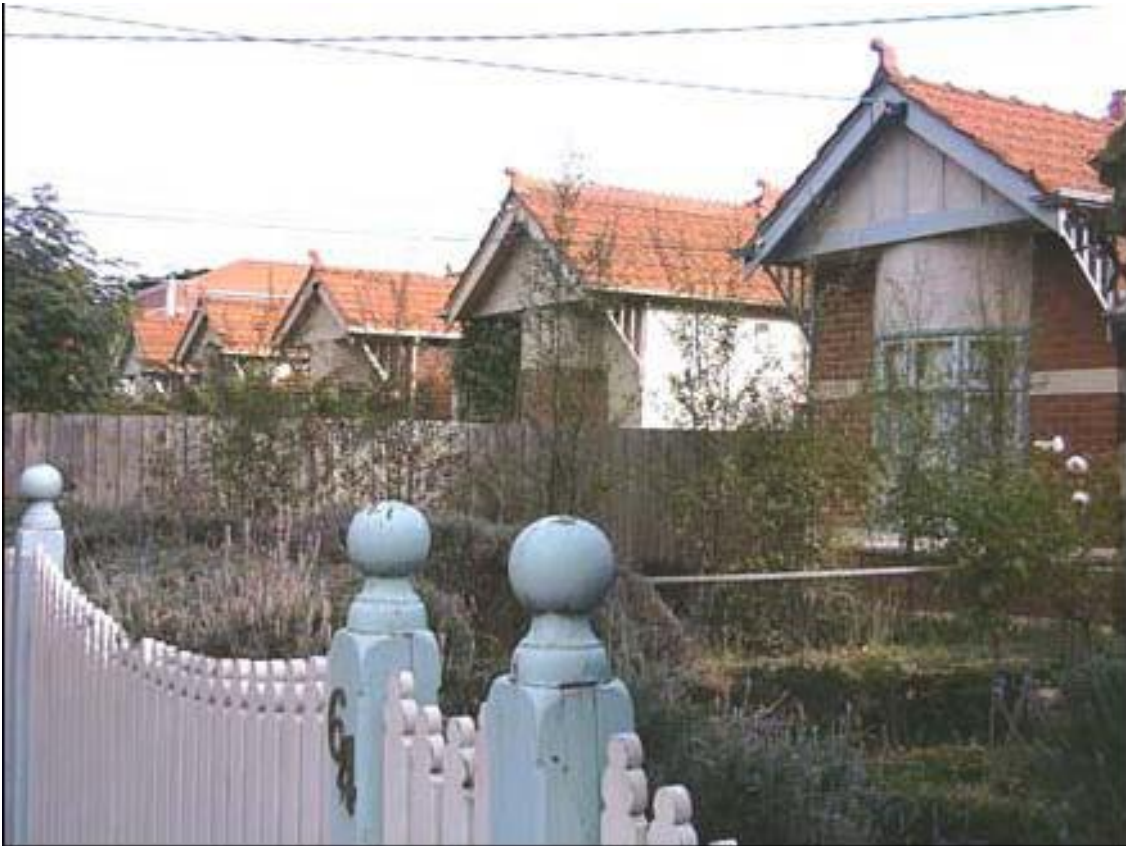
Figure 6.27-1 – Typical row of semi-detached Queen Anne Revival housing in Ruskin Street
