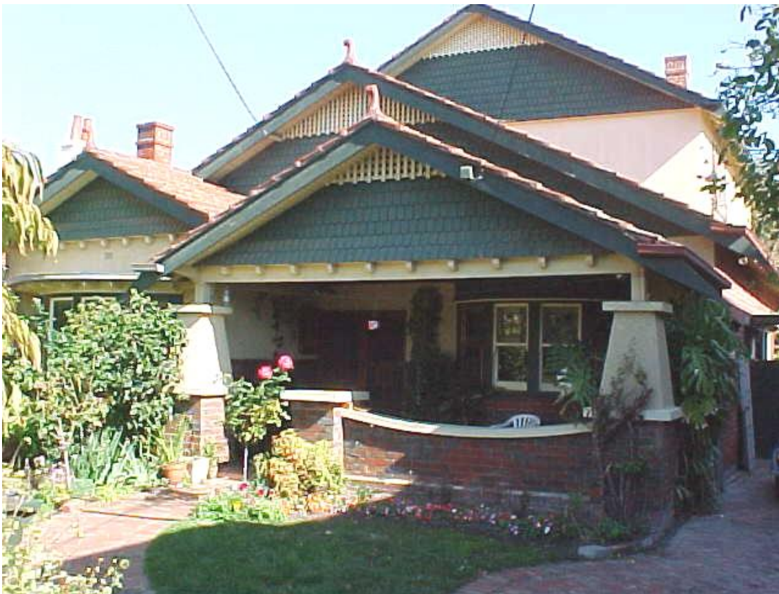
Figure 6.25-5 – Typical 1920s bungalow – Orange Grove, East St Kilda
