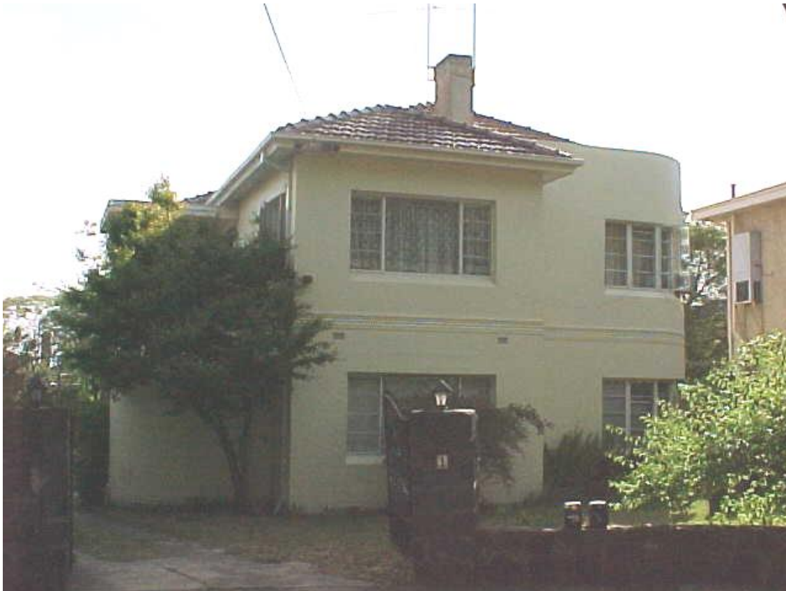
Figure 6.21-3 – Flats, No 1 Holroyd Court (c.1938)
