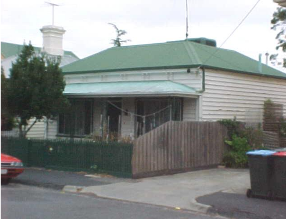
Figure 6.18–5 – Double fronted house at No 25 Chusan Street, East St Kilda
