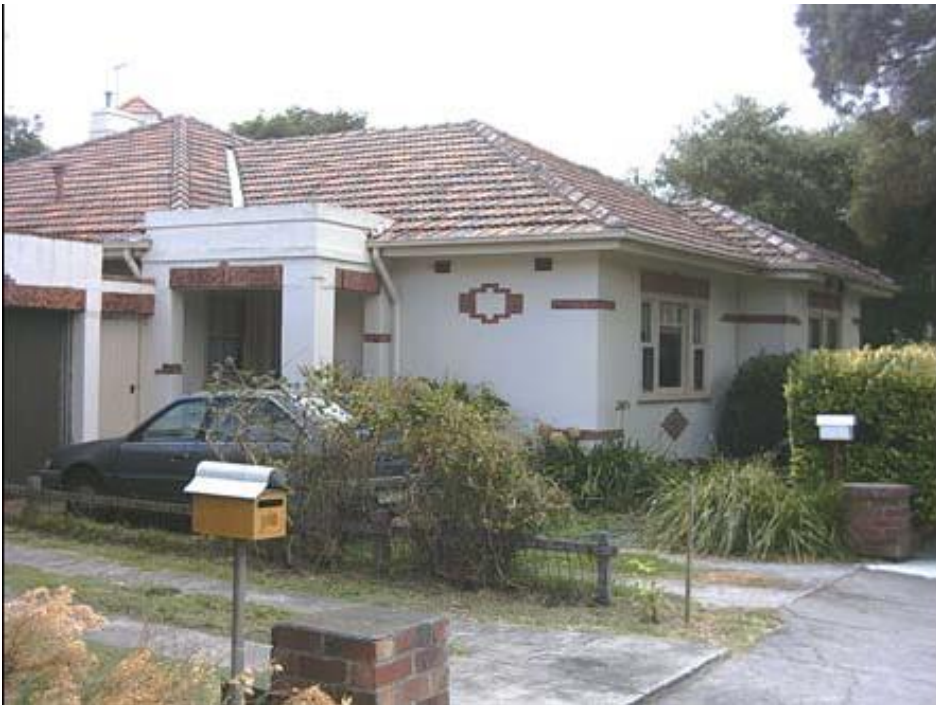
Figure 6.29-4 – Typical pair at 3 – 5 McCrae Street, note: garage and low woven-wire fence.
