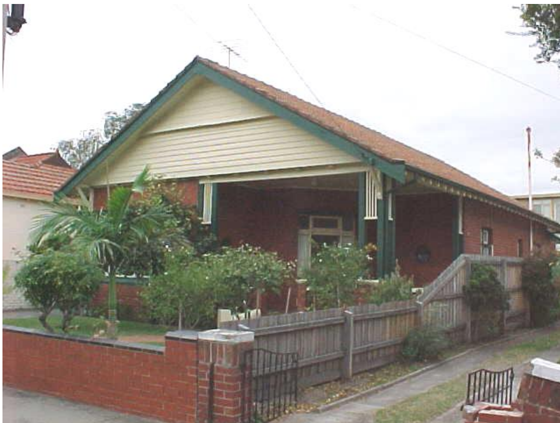
Figure 6.22–6 – Bungalow-style house at No. 8 Kalymna Grove, East St Kilda
