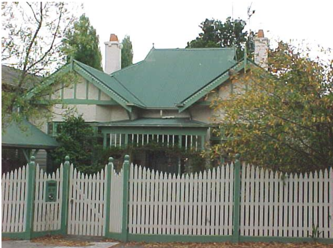
Figure 6.22–5 – Weatherboard house at No. 27 Kalymna Grove, East St Kilda
