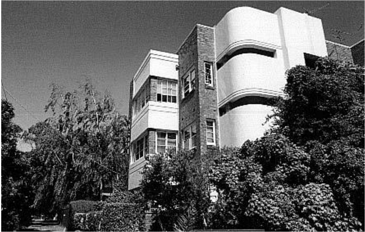
Figure 6.16-1 – “Taradale” at no. 229 Brighton Road defines the northern extremity of the Area.
