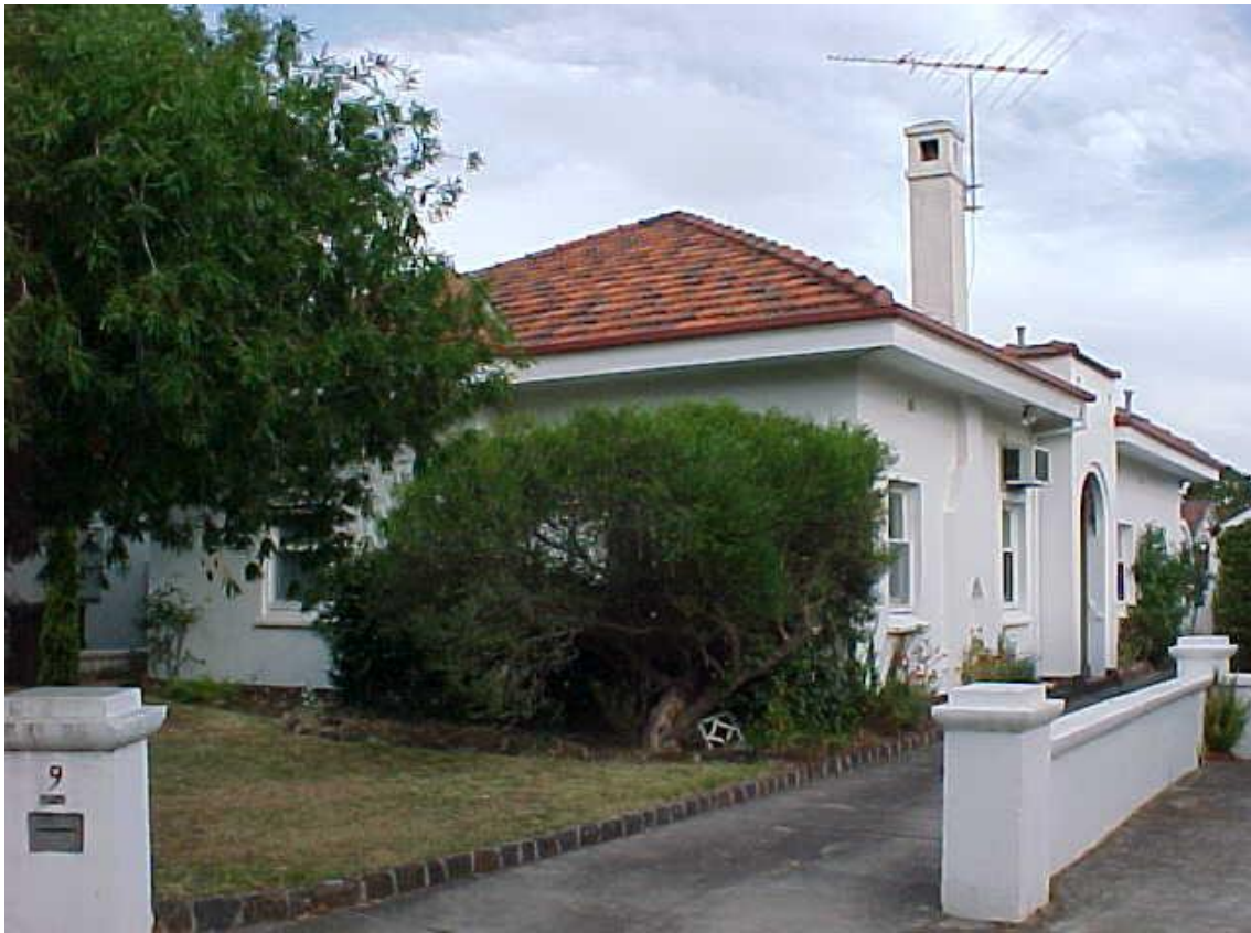
Figure 6.23-4 – House at Mooltan Avenue (1928)
