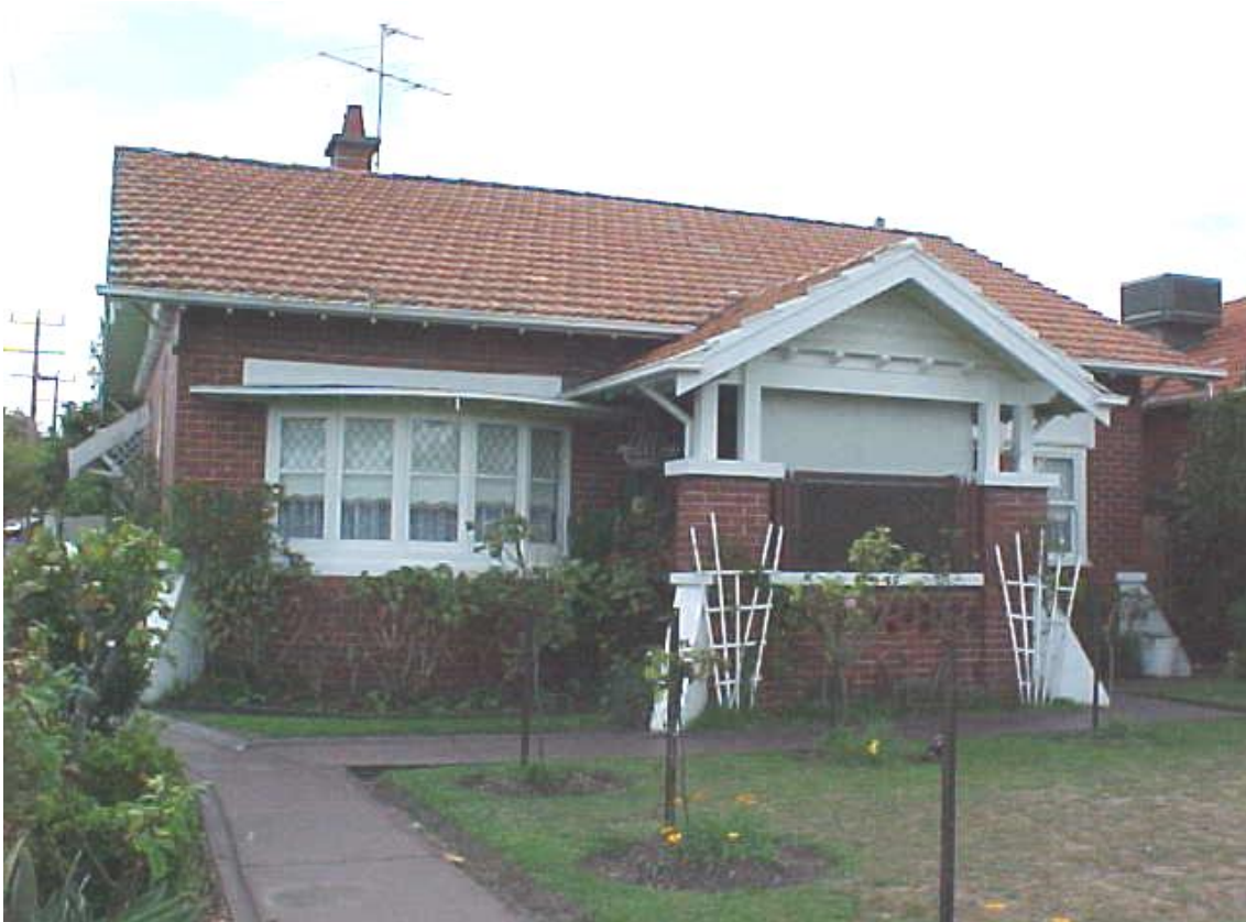
Figure 6.24-2 – Bungalow – 160 Alma Road (c.1925)
