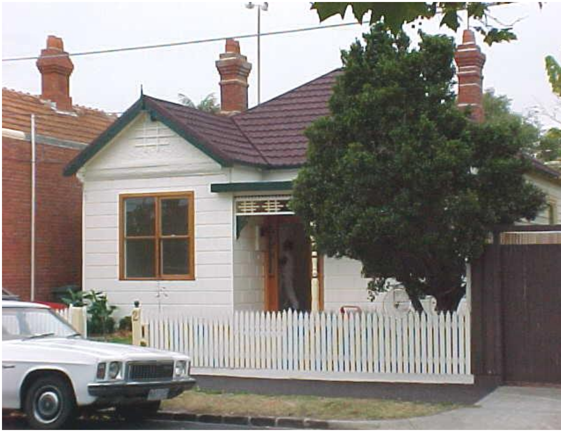
Figure 6.19-4 – Weatherboard House at No. 2
