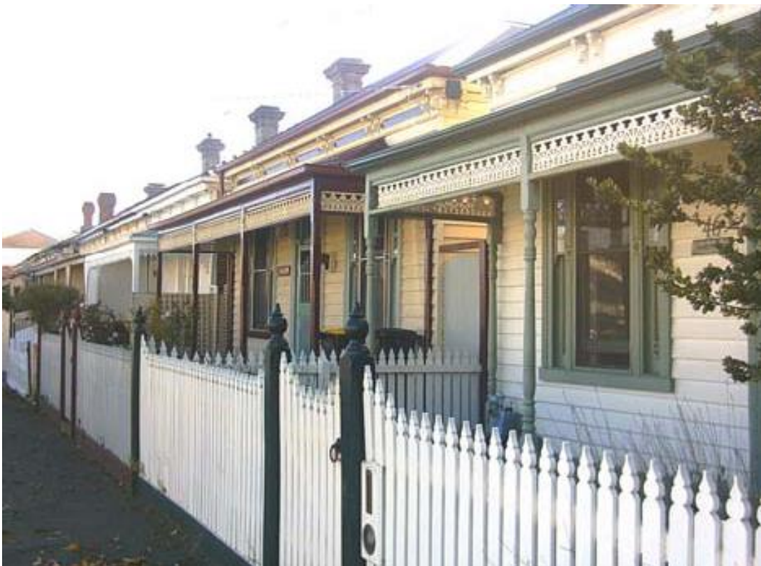
Figure 6.30-8 – Row of three speculative double-fronted Boom-style timber villas at 44-48 Nightingale Street
