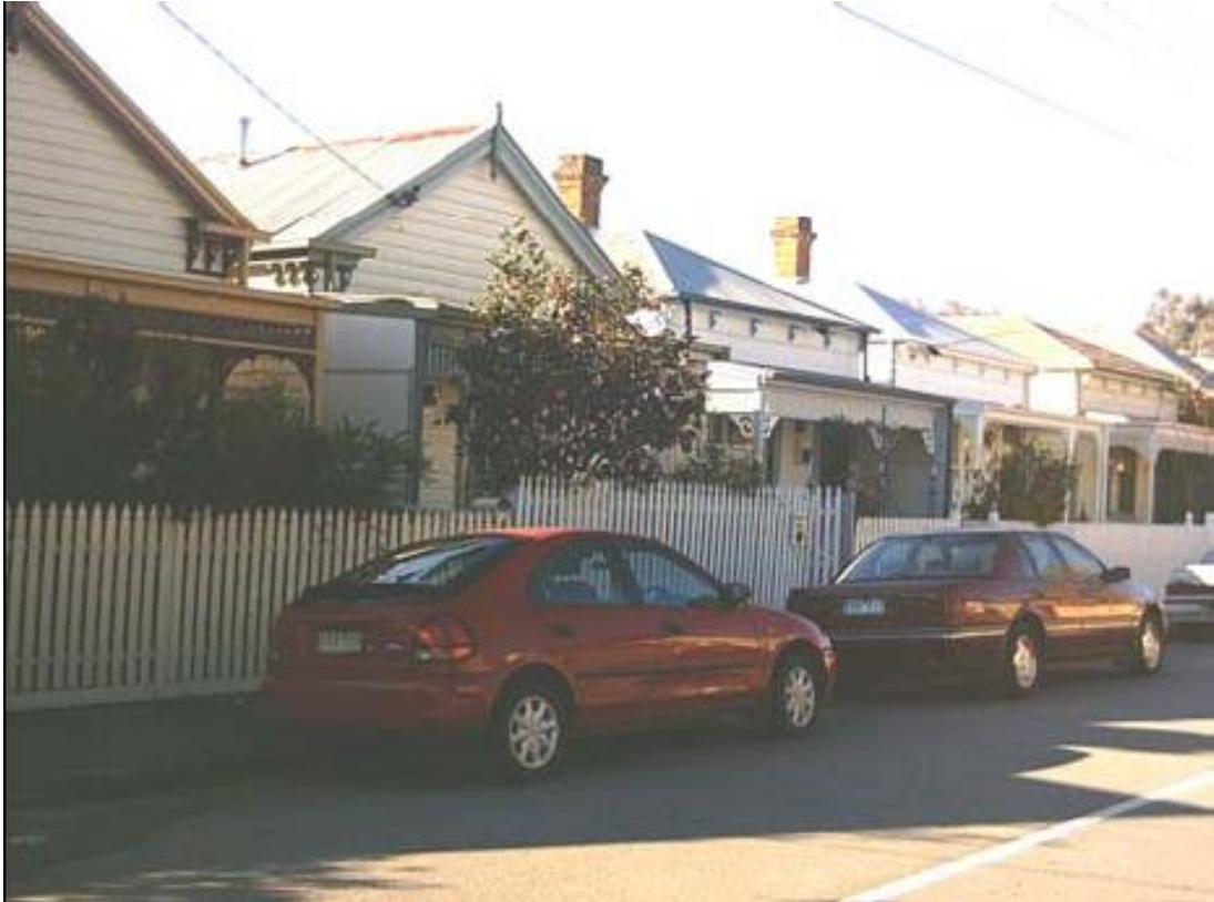
Figure 6.30-5 – Mix of gable-ended and hip-roofed single-fronted timber cottages on north side of Rosamund Street
