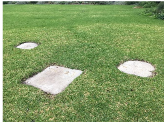
Figure 25: An example of the multiple underground services that run through the green spaces within the central portion of the study area_23/04/20
