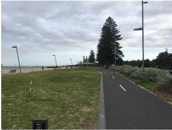
Figure 16: General view of the Elwood foreshore area, showing landscaping and the construction of walking paths and lamp posts, facing north_23/04/20
