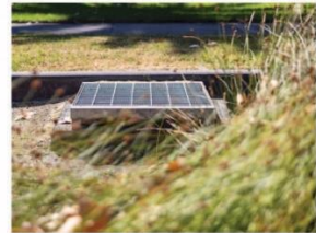
Green infrastructure – roofs, walls, WSUD
