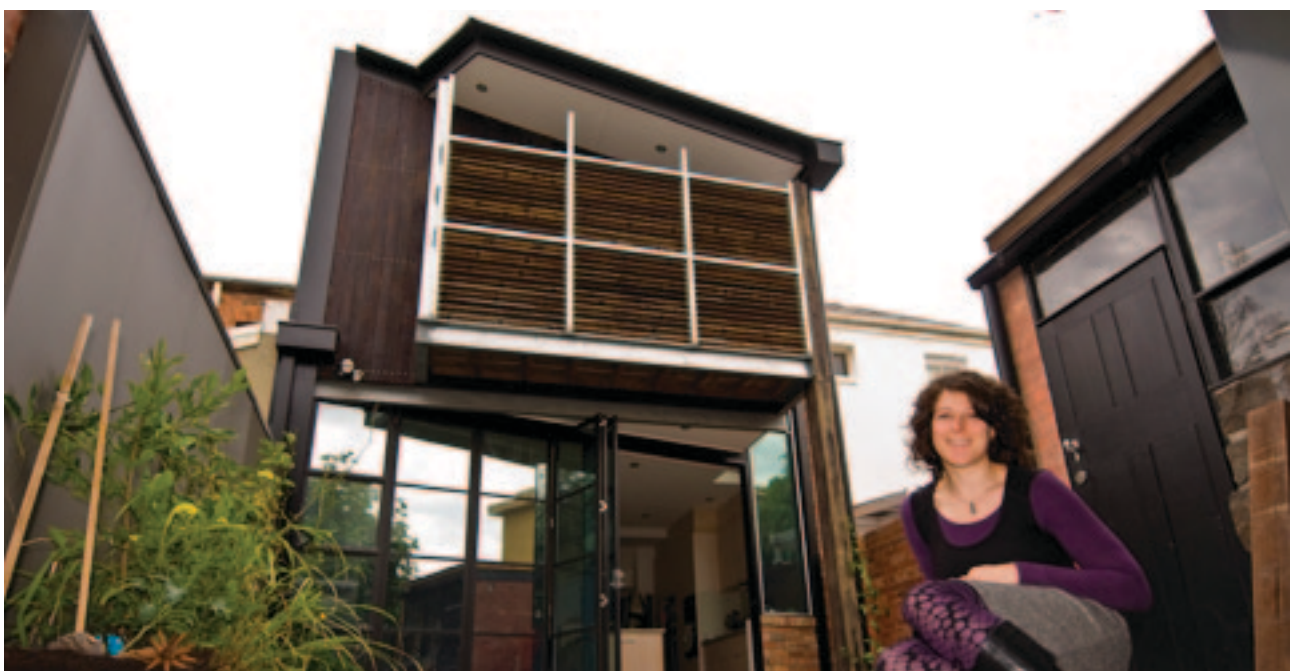
This traditional terrace in Albert Park now has triple glazing, deep eaves and uses passive solar design. The result – a truly comfortable and low carbon home!
