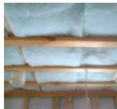
Insulation helps to make a building more thermally efficient so it gains and loses less heat
