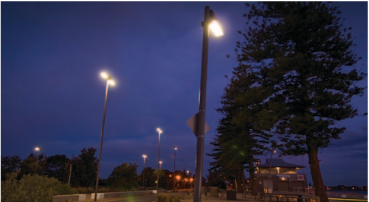
Council has started to retrofit its public and street lights with much more energy efficient alternatives
