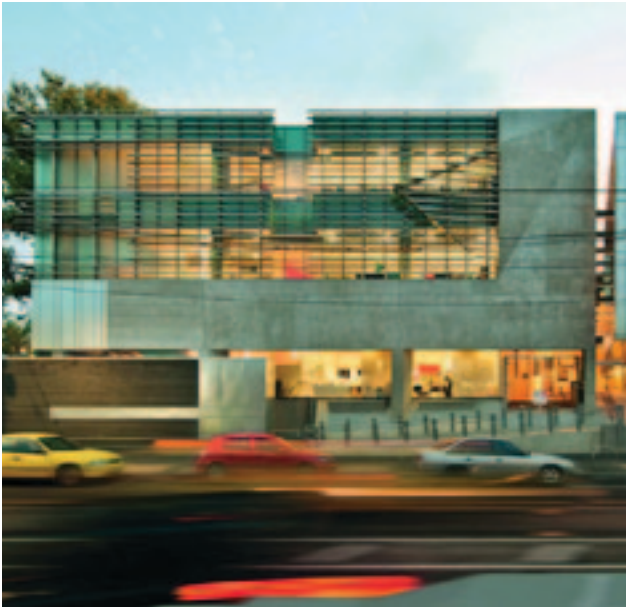
St Kilda Town Hall, above, is Council's largest building and highest energy using site.
