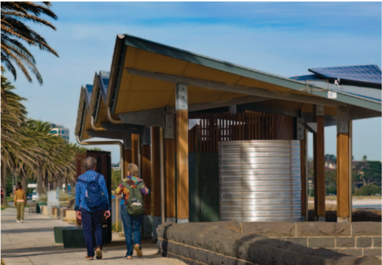
The public washroom at Middle Park Beach collects its own solar power and rainwater
