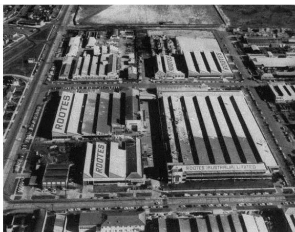
Figure 1 – Rootes factory in 1950s looking west, showing recent extensions with light roofs (Source: The Supreme Sunbeam)
