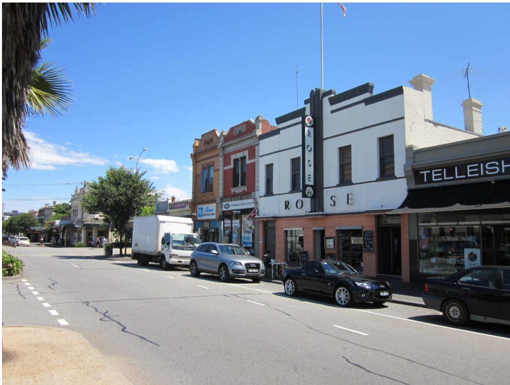
Figure 6.5–3 – View of the west side of Bay Street
