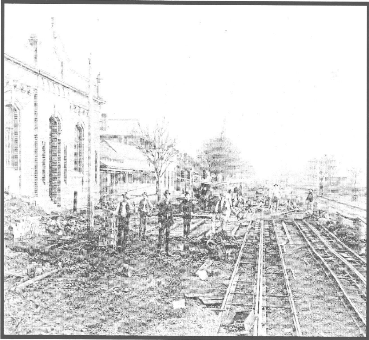
Figure 6.8-3 – City Road in 1890, showing the cable tramway being installed with the engine house at left. Notice the absence of development on the right hand side of City Road.
