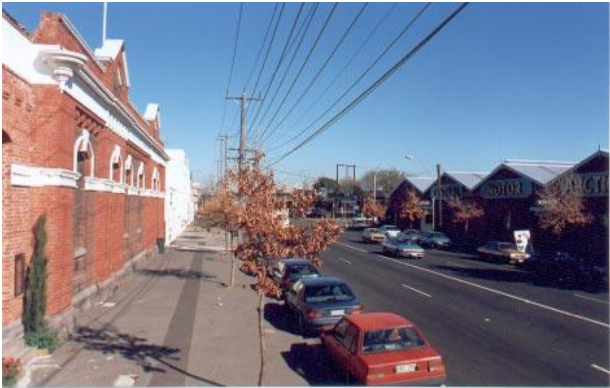
Figure 6.8–5 – City Road, with the former cable tramway engine house at left and the former Johns and Waygood factory at right.
