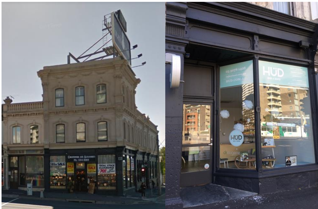
Figure 6.10-19 – 140-146 St Kilda Road, with one of the original shopfronts at right
