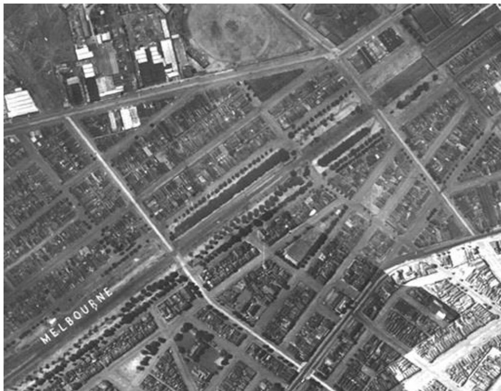
Figure 6.3-5 – 1945 Aerial showing the intersection of Williamstown Road and Inglis Street.
