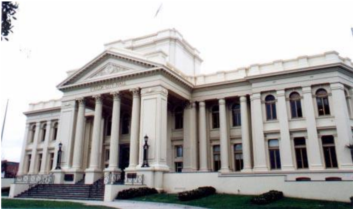
Figure 6.11-8 – The St. Kilda City Hall dominates the Carlisle Street/Brighton Road intersection and forms a group of public buildings with the St. Kilda School and the Holy Trinity Anglican church
