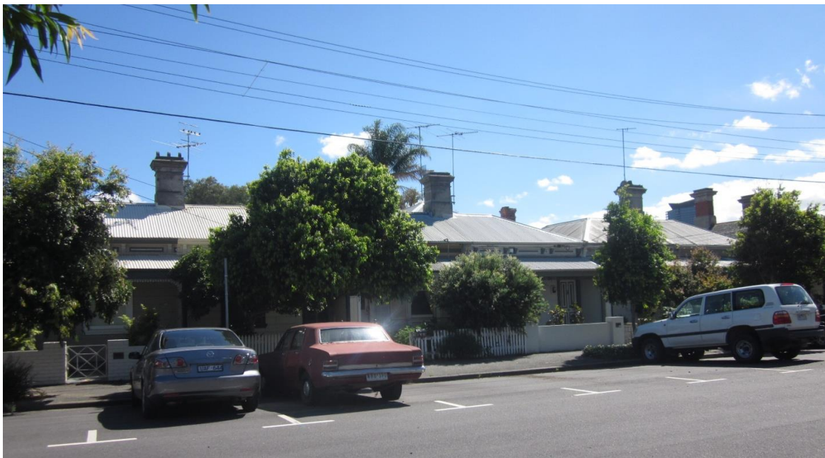
Figure 6.3–7 – Paired timber villas in Ross Street, north of Bridge Street with central rendered brick chimneys.
