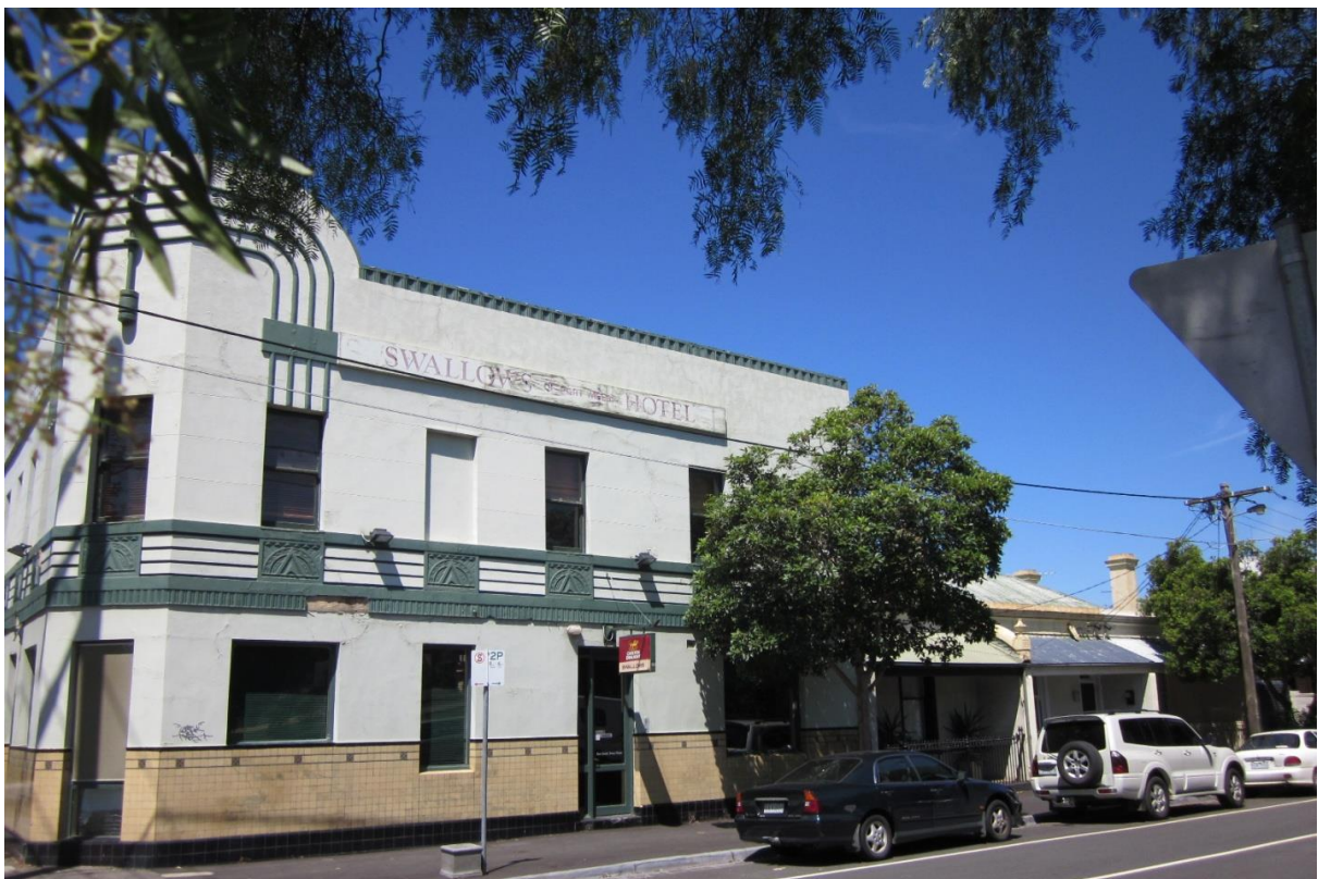
Figure 6.6–7 – Swallows Hotel, corner Ingles and Station Streets.
