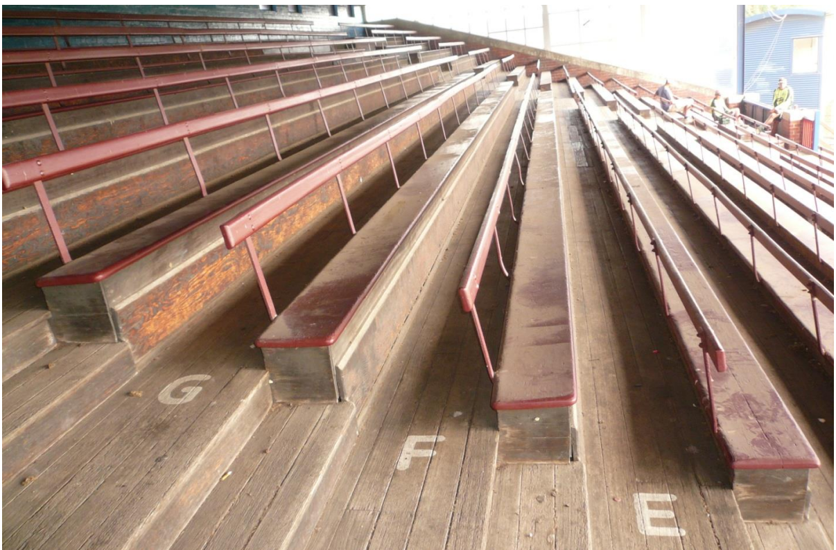
Figure 6.38-5 – Timber seating plats and painted row identifiers.
