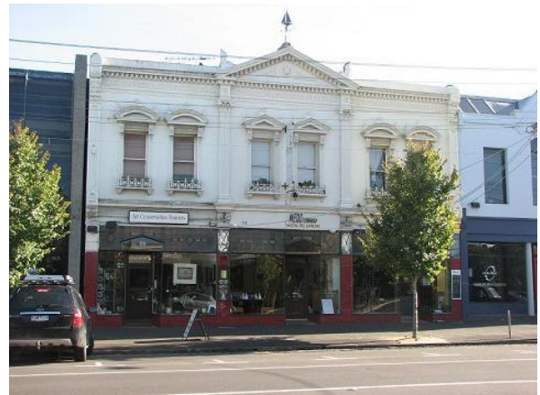
Figure 6.34-6 – Group of three residential shops in Bridport Street, showing original shopfronts at ground floor
