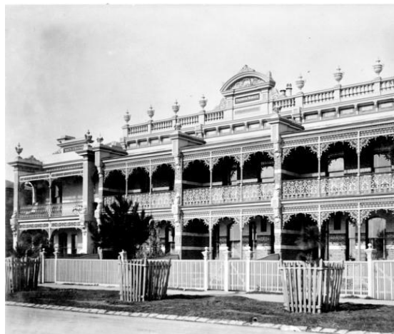
Figure 6.35-4 – 1889 photograph by David Wood, showing then recently-completed terrace houses at 62-65 Canterbury Road
