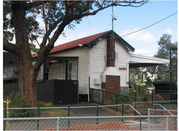
Figure 6.37-9 – The former Middle Park Railway Station (now a café) on the western edge of the park
