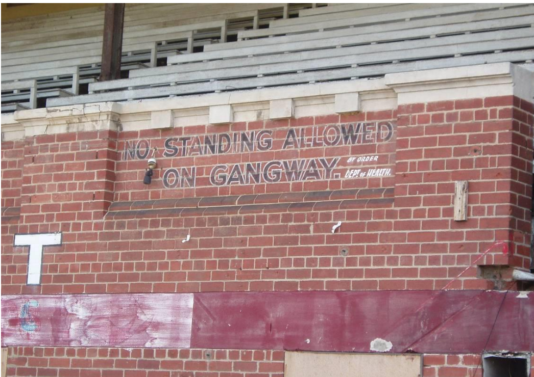
Figure 6.38-9 – South Melbourne Grandstand, showing early painted signage and original timber seating.
