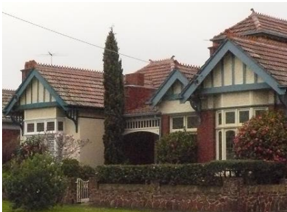
Figure 6.35-16 – Edwardian red brick villas, McGreggor Street
