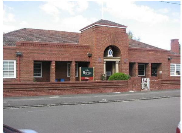
Figure 6.37-11 – The former military drill hall (1935), on the park's northern edge
