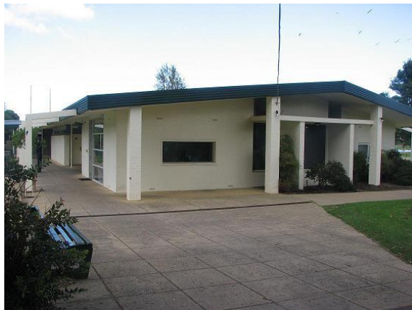
Figure 6.37-12 – The golf course building (1960), which once included the celebrated Rob's Drive-in Restaurant
