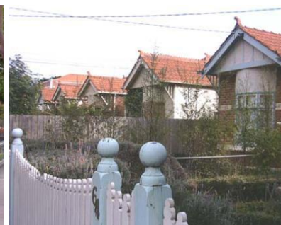
Figure 6.35-21 – Row of Edwardian red brick villas in Ruskin Street, Elwood
