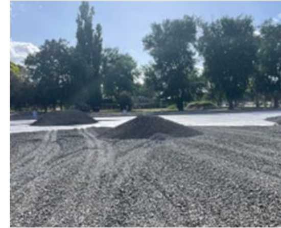
JL Murphy (Pitch 2) - drainage and rock installation
