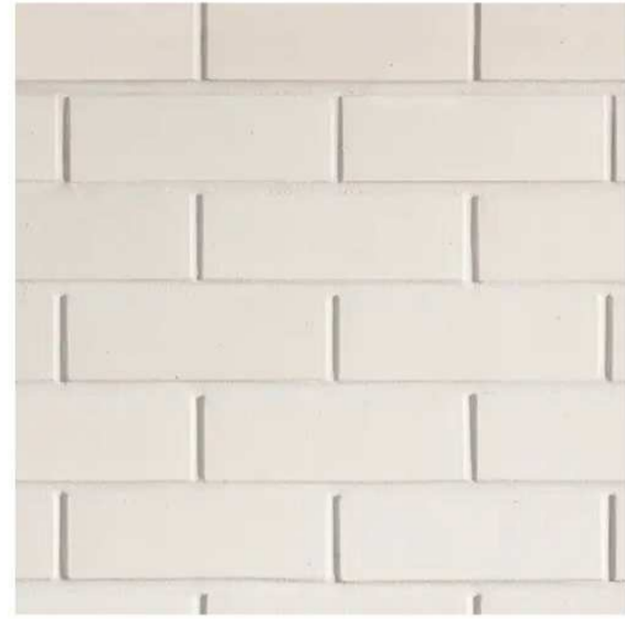
CODE: BRK1 MATERIAL: BRICK WORK FINISH: WHITE BRICK WITH COLOUR MATCHED MORTER LOCATION: EXTERNAL WALLS AS INDICATED
