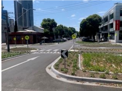
Raingarden and intersection improvements at Market and Clarke Streets South Melbourne
