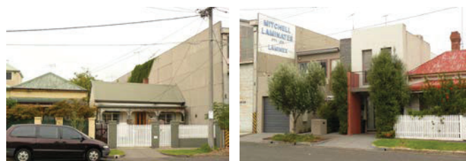
Above: south side of Garton Street.
