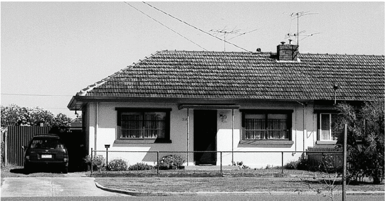
Figure 5. One of the most intact early concrete dwellings, 350 Howe Parade, Fishermans Bend Estate.
