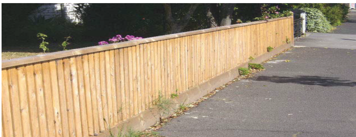
Figure 19: Timber fence of simple board pickets with a top rail (acceptable)
