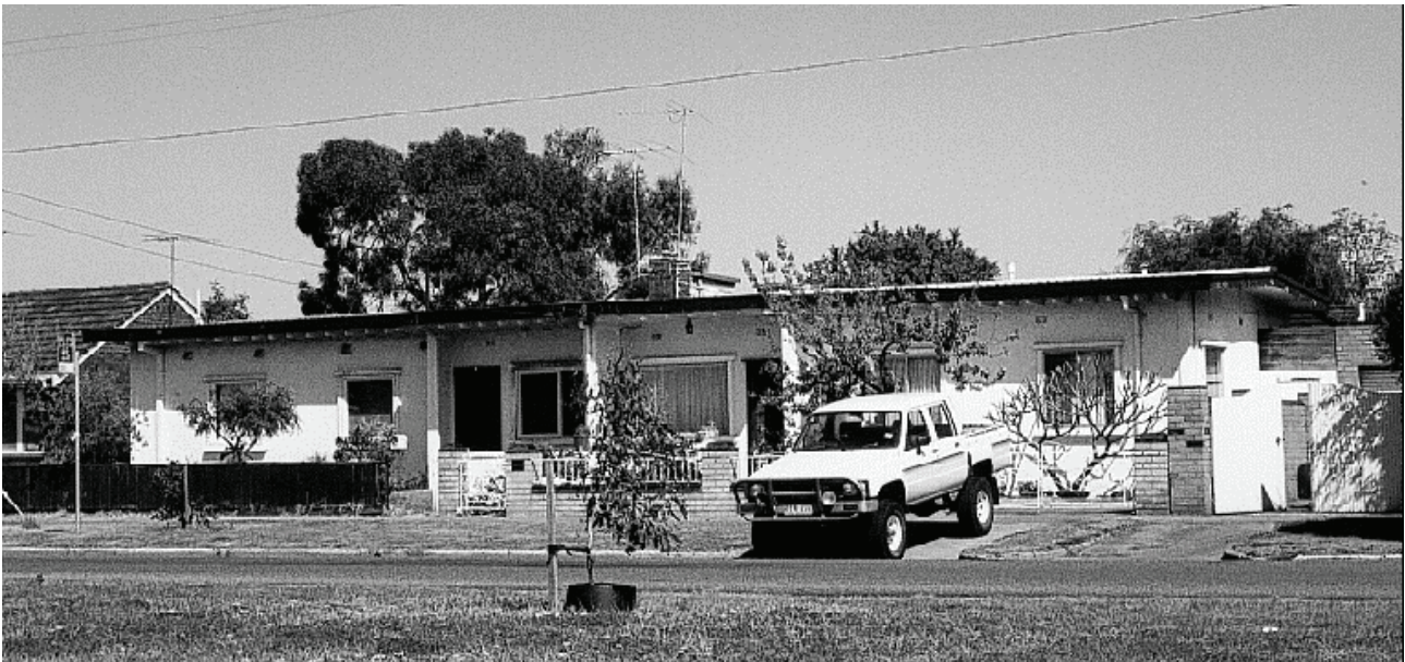
Figure 4 The first experimental dwellings using the TW Fowler system of concrete prefabrication, 324-326 Howe Parade, Fishermans Bend Estate.
