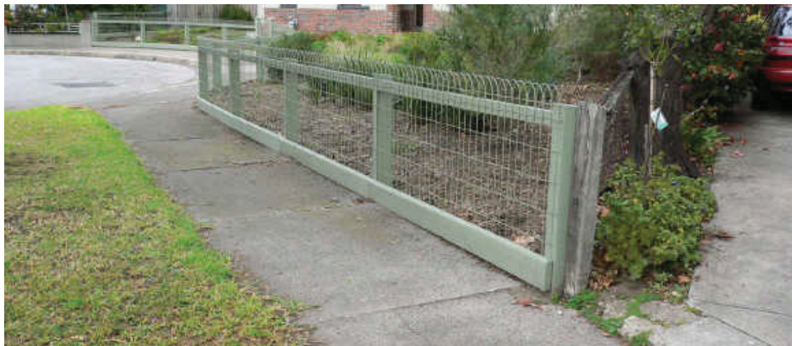
Figure 18: New woven wire fence on timber framing set to a low height (acceptable)
