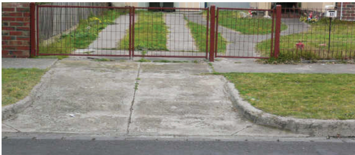
Figure 24: Driveway and pedestrian pathways as plain uncoloured concrete tracks, causing minimal use of hard pavings.
