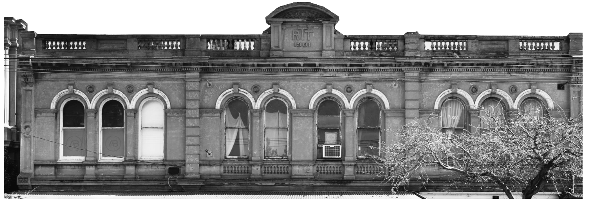
Existing Heritage Facade at 146-150 Bridport Street
