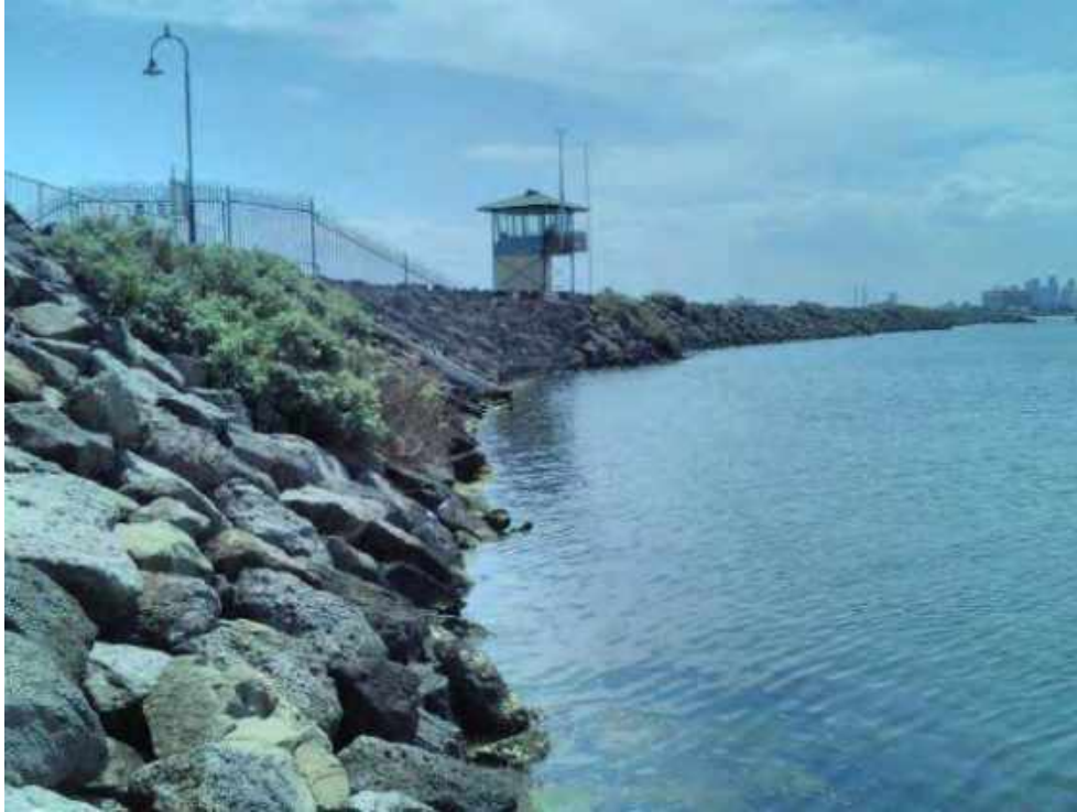
Plate 29. St Kilda Breakwater
