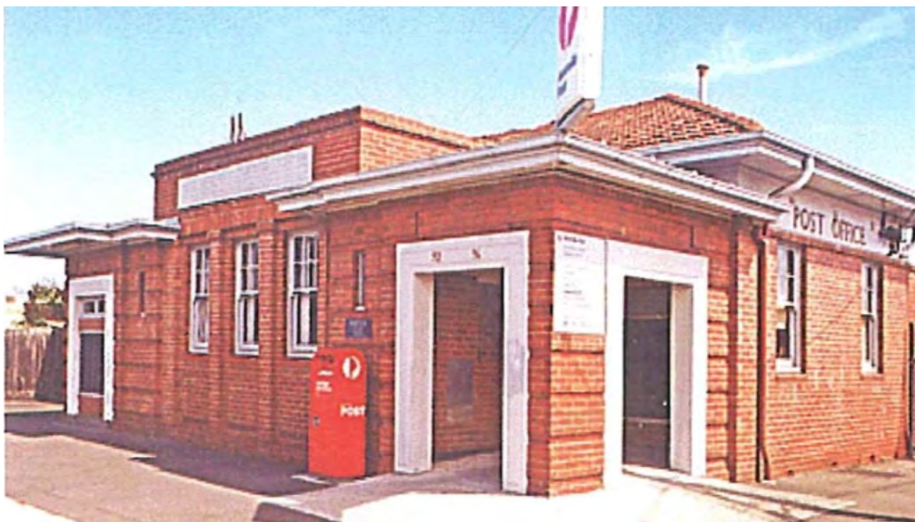
Figure 26. Fairfield Post Office. (City of Darebin, 2001)
