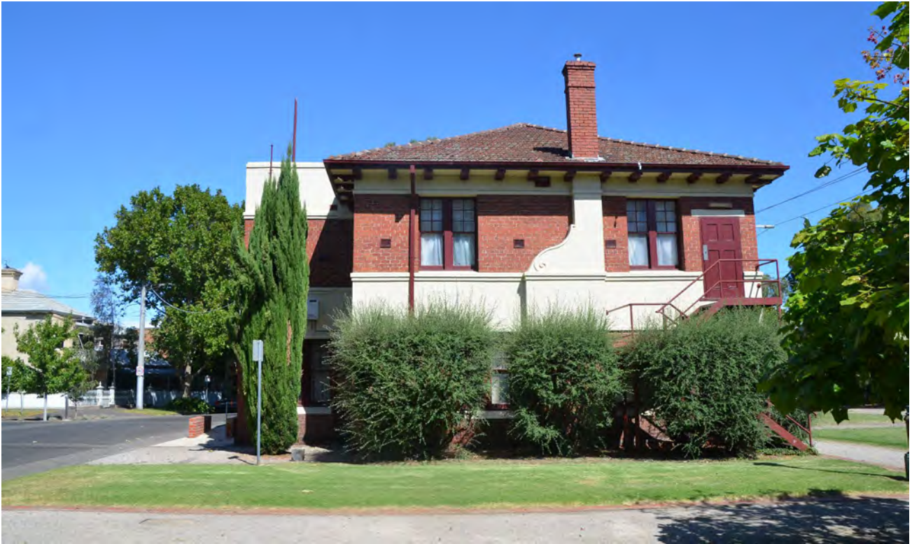
Figure 3. North elevation, exterior – note original scroll detailing to the external chimney breast and modern metal egress stair.
