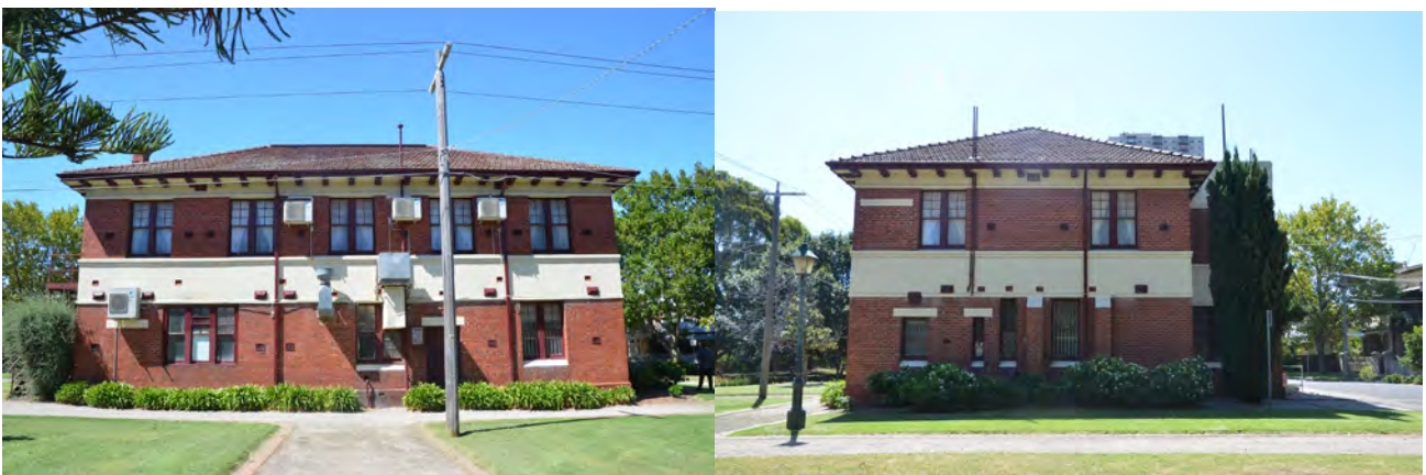
Figure 4. West elevation (left) & south elevation (right); note significant building plant on west elevation.
