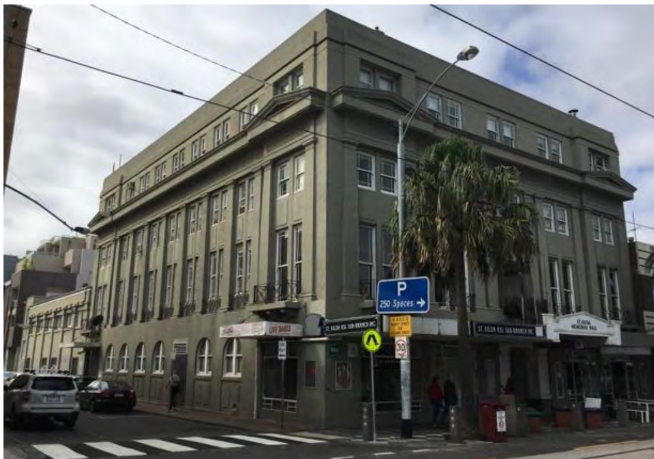
Figure 19. St Kilda Memorial Hall, 1923-24. (City of Port Phillip, 2017)
