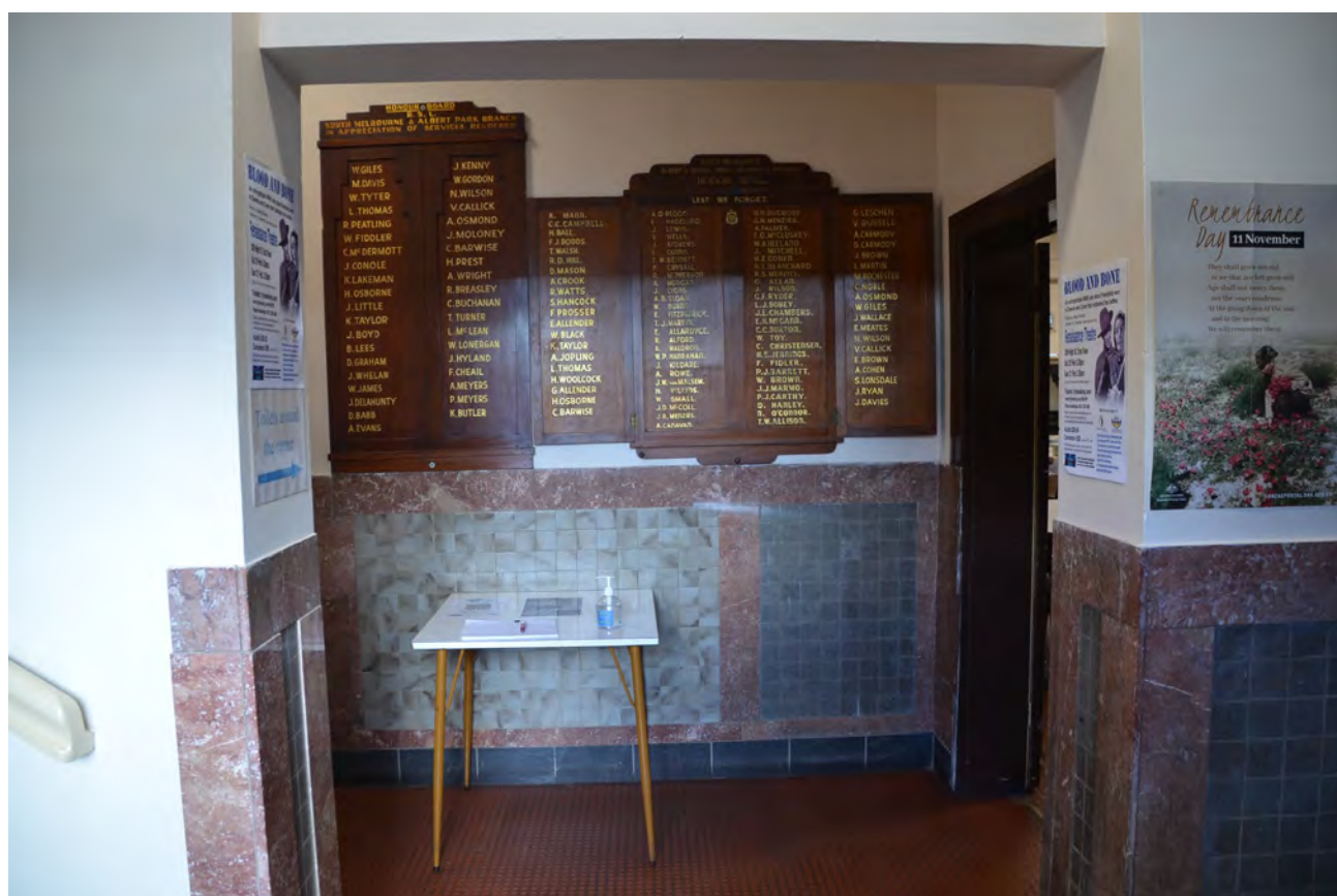
Figure 5. Main entry, interior – original Alicante marble and tile dado with WWI and WWII honour boards above
