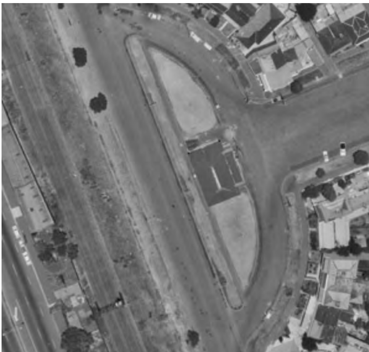
Figure 17. The Memorial Hall in 1971. Note the loss of all trees on the reserve, and the continued presence of Ferrars Place to the rear. Only one external staircase remains, on the north side of the building. (Landata)
