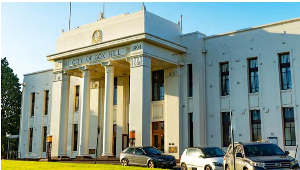
Figure 31. Box Hill Town Hall. ( www.boxhilltownhall.com.au , n.d.)
