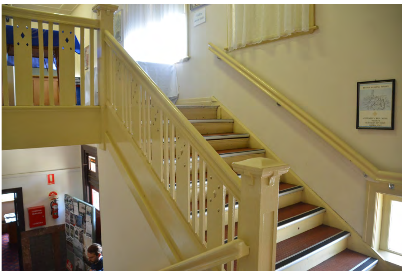
Figure 7. Staircase, interior – highly intact, although over painting diminishes their appearance
