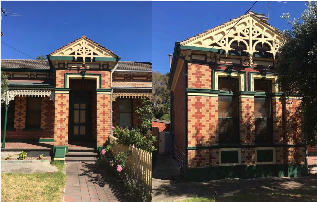
Porch and south gable of nos. 29-31
