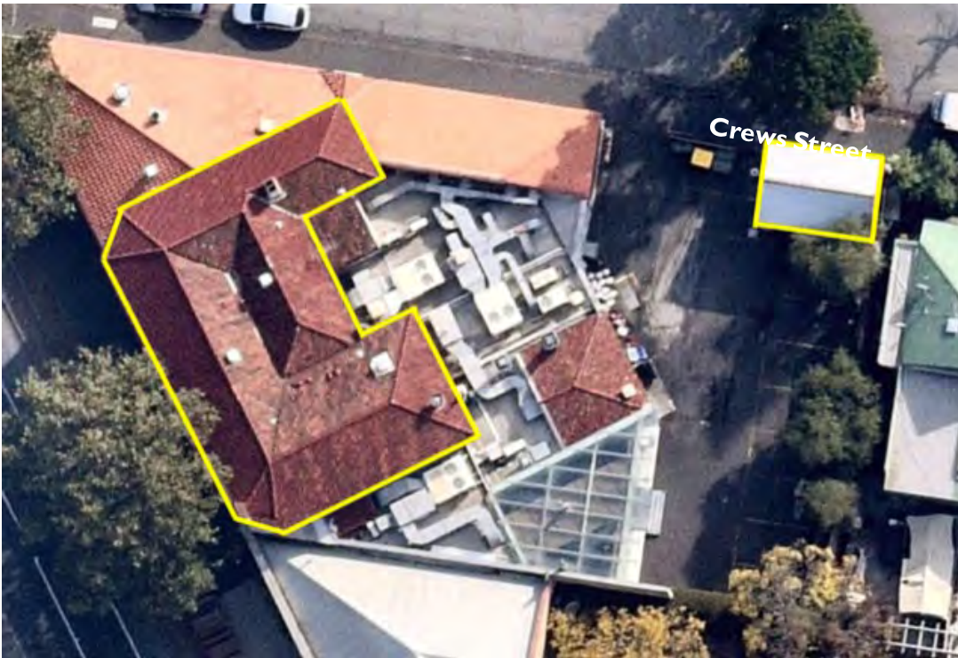
Figure 3: Aerial, showing contributory buildings outlined in yellow (Source: Nearmap.com).
