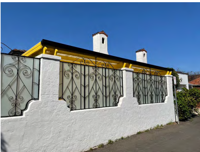
The original rendered piers of the side pergola and two of the 'dovecote' chimneys
