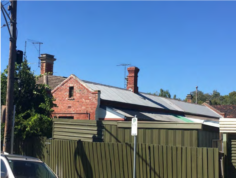
Rear gabled wing of nos. 29-31.
