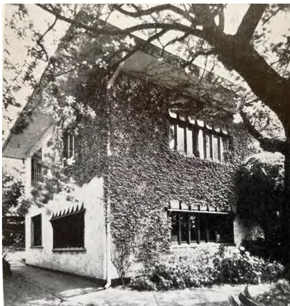
Figure 2: Inglesby – note the horizontal windows with expressed mullions and shallow hoods (Source: Edquist 2008:39)
