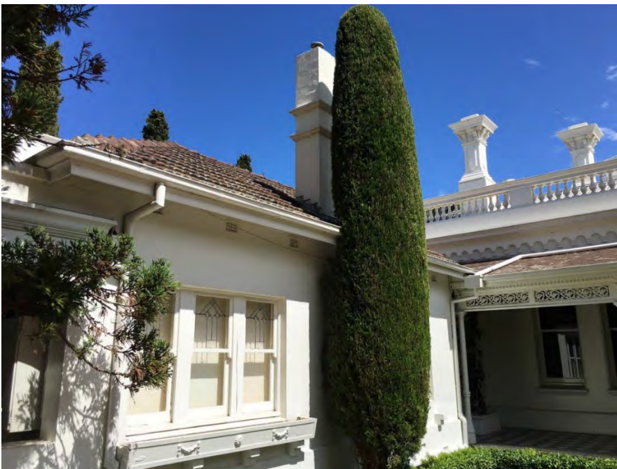
The 1935 addition at the south end of the east elevation
