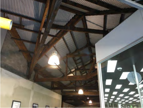
Internal roof trusses within former car shed
