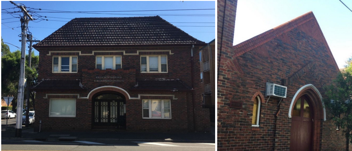
Figure 8 – The former Joseph Allison Funeral Parlour at 362A Carlisle Street (front elevation to Carlisle Street at left and former chapel facing Balston Street at right)
