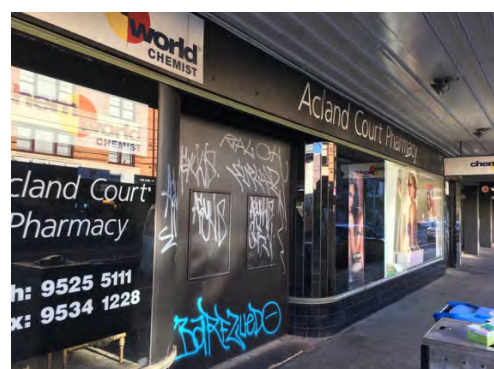
Barkly Street elevation and shopfront
