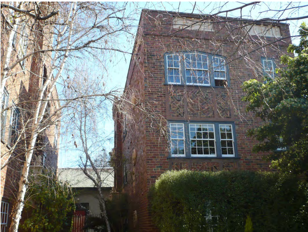
Main elevation of the north block
