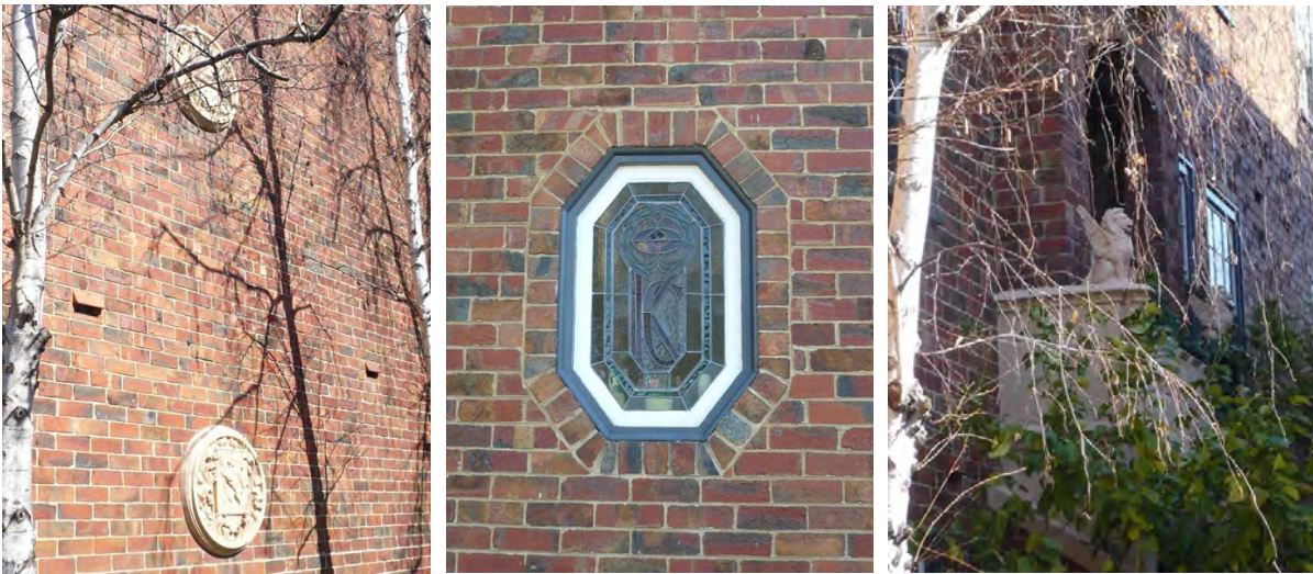
Building details from left: Medallions with heraldic symbols; octagonal leadlight glass window with pattern featuring an interlocked 'K' and 'C' in Gothic script; rendered balcony above entry to stairwell with Griffins in front of arched opening
