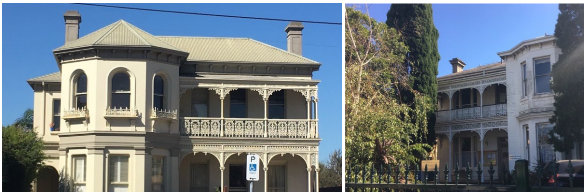
Figure 4 – Victorian Italianate villas at 307 (left) and 366 (right) Carlisle Street
