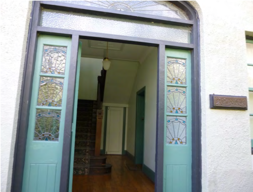
Entry to rear two-storey wing with arched leadlight fan light and sidelights, and original staircase
