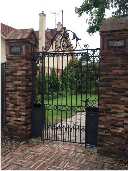
Original pedestrian entry gates.
