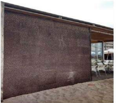
Cork facade panelling
