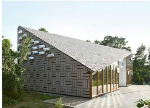
Habitat boxes and timber/cork panelling
