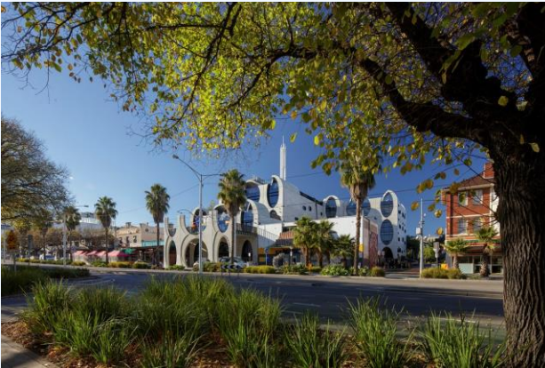
The Victorian Pride Centre was commended for its sustainable design as part of Council's recent Design and Development Awards.
