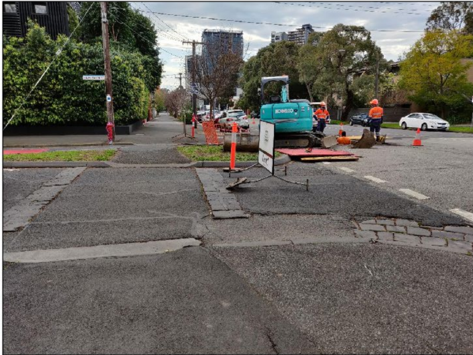
Photo 6: Park Street at Eastern Road intersection, facing east
