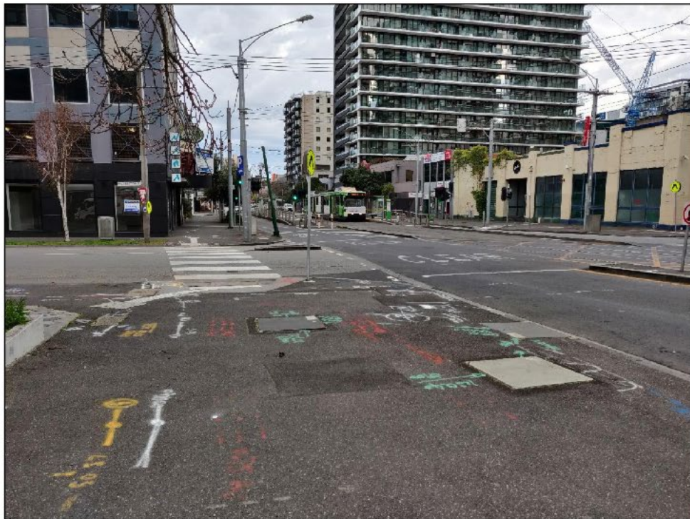
Photo 4: Park Street at Palmerston Crescent intersection, facing west
