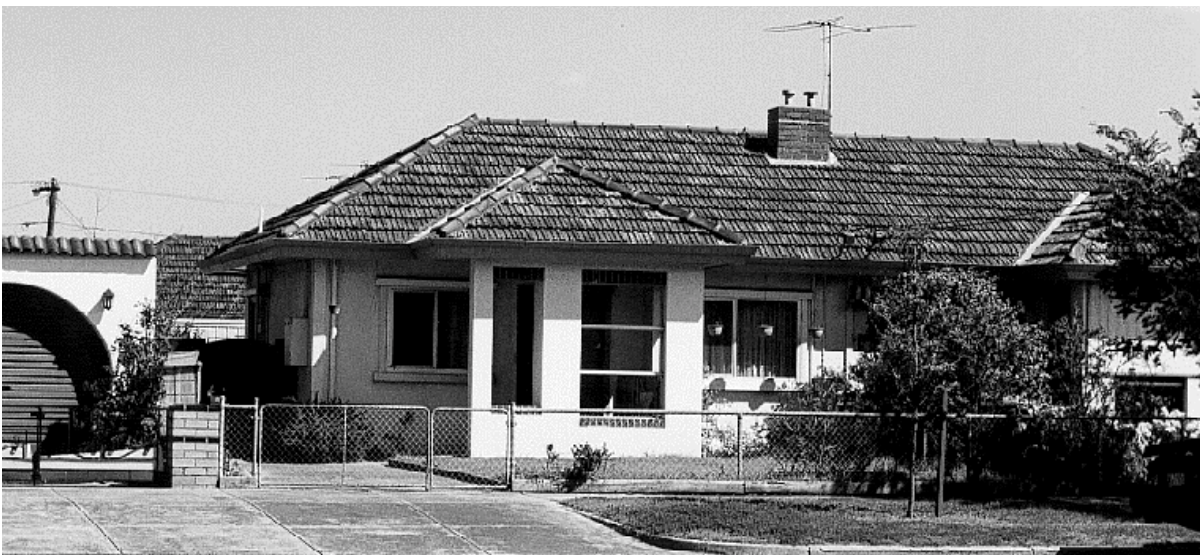
Figure 26. Later rendered brick porches on concrete dwellings.
