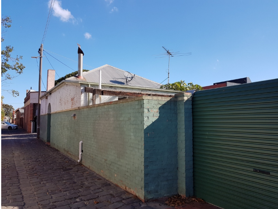
Figure 3 The east and north elevations of the subject property. The side fence and roller door are also visible.
