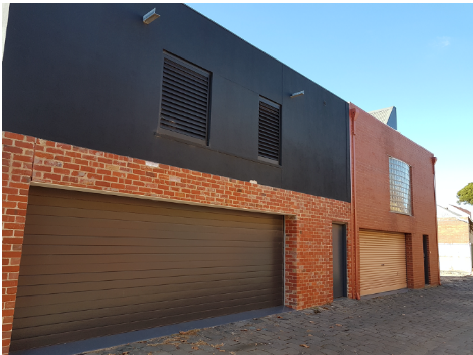
Figure 7 Modern outbuildings to the rear of 202 and 204 Page Street, west of the subject site.
