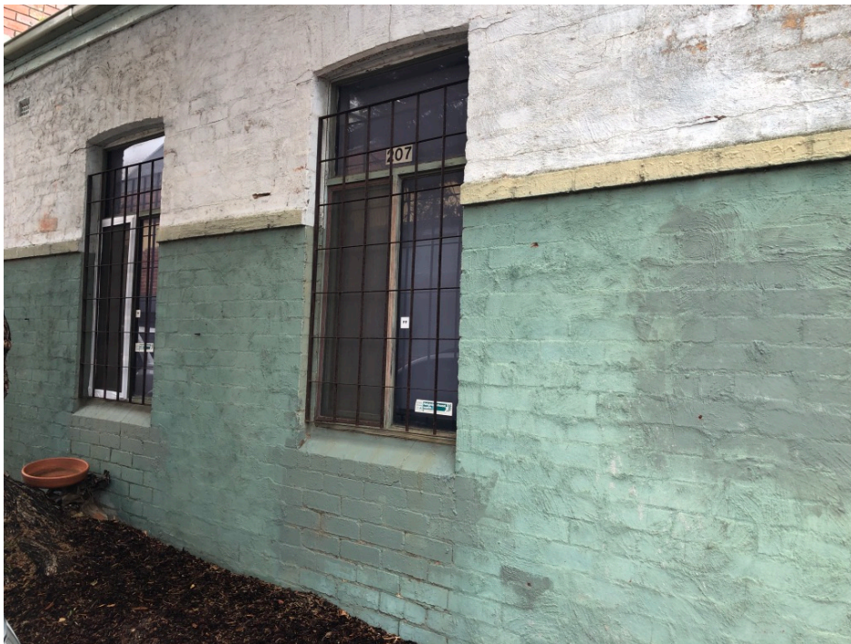
Figure 4 The southwest elevation of the subject property. These two windows appear to have been altered in the period since the building was bagged and painted.
