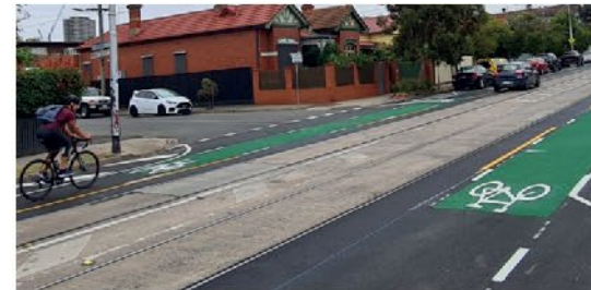
Chapel Street with green pavement marking with bike lane and painted islands.
