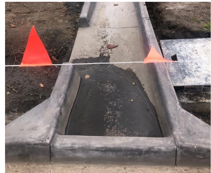
Passive Irrigation system for median tree planting in Albert Road (source CoPP)
